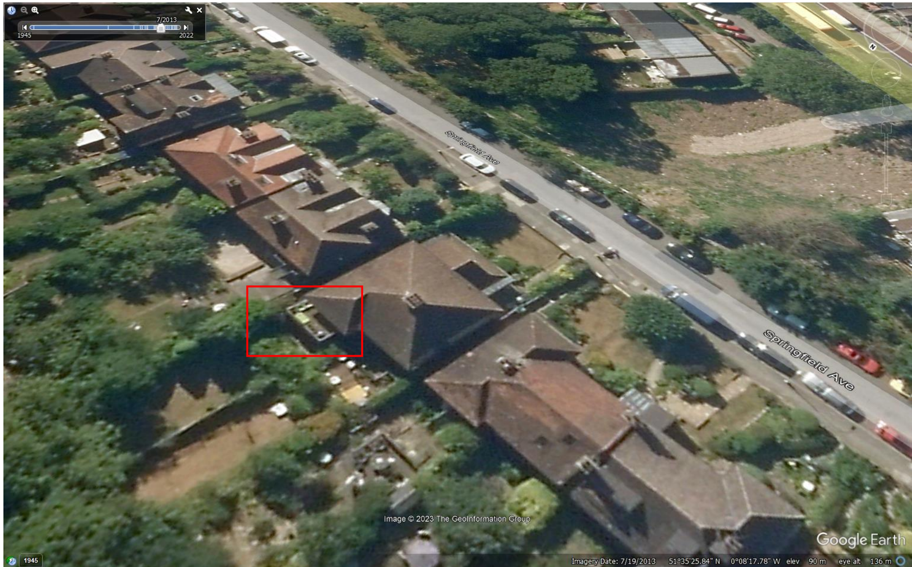
Google Earth satellite image showing roof terrace 19 July 2013 (dated lower right)
