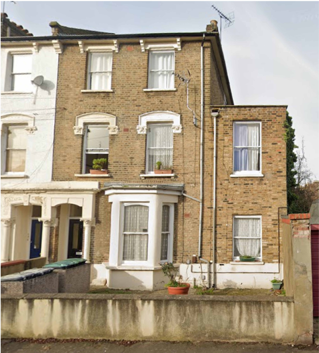
FRONT ELEVATION PHOTOGRAPH
