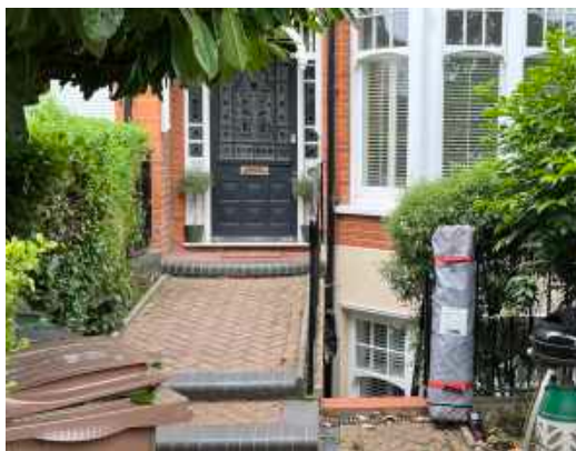
No. 30 Grand Avenue front lightwell
