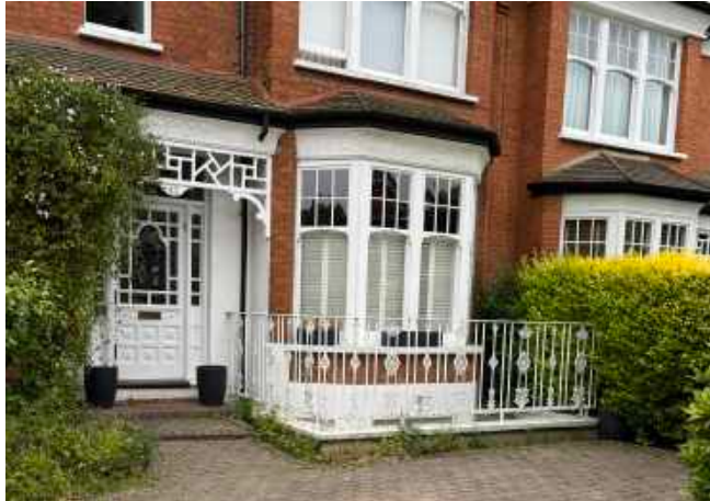
No. 42 Grand Avenue front lightwell
