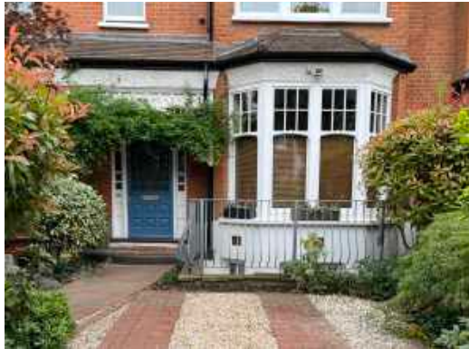
No. 26 Grand Avenue front lightwell
