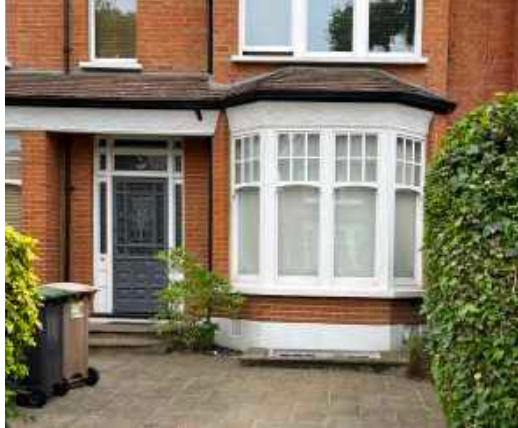
No. 18 Grand Avenue front lightwell
