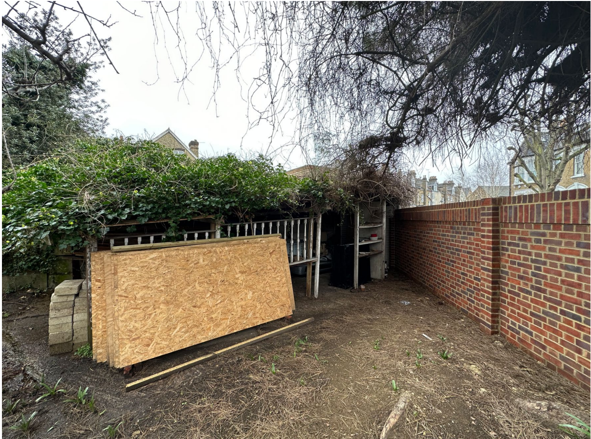
Photo showing the existing garage structure.
