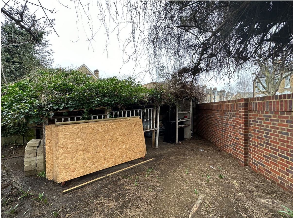
Photo showing the existing garage structure.
