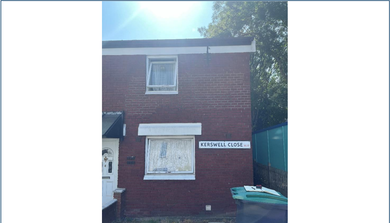
Photo 01 Existing Front Elevation
