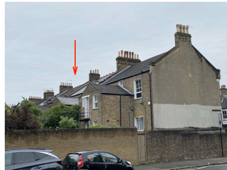
VIEW FROM FERME PARK ROAD
