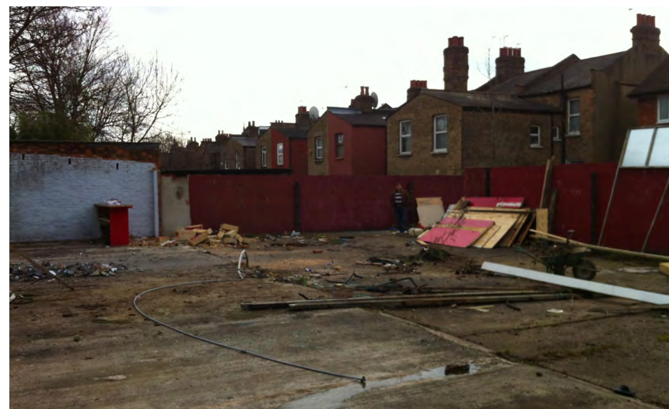
20. Photo 2 - South East view of the site, showing the rear of the Victorian Houses on Effingham Road
