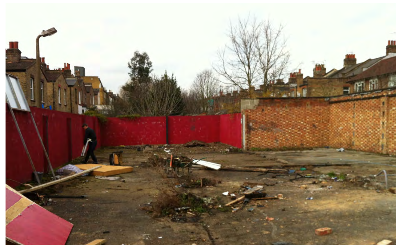
19. Photo 1 - West view of the site, showing existing boundary wall
