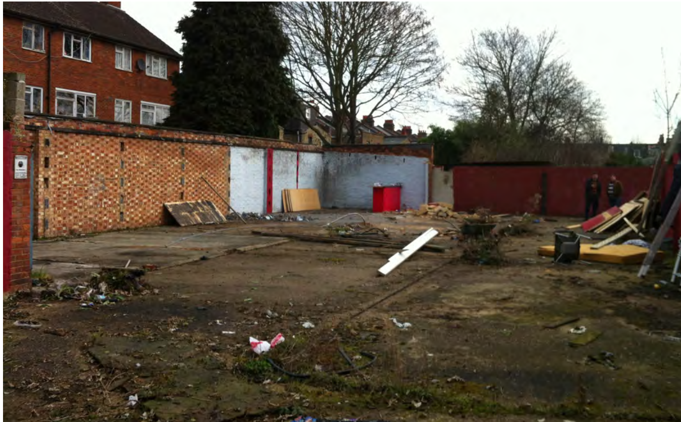
21. Photo 3 - North East view of site, showing existing boundary wall
