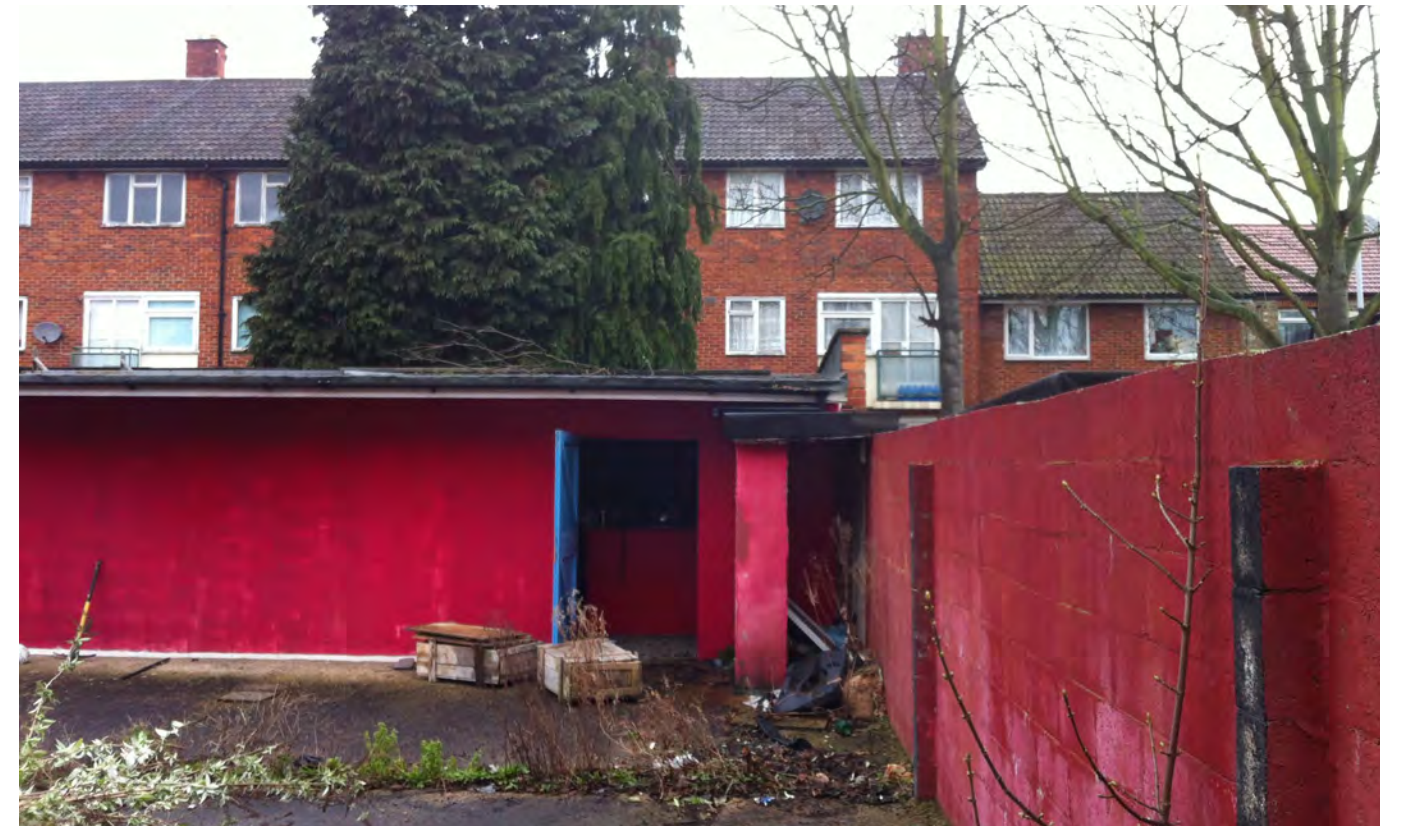
29. Photo 11 - View of previous shed that has now been removed from the North East corner of the site
