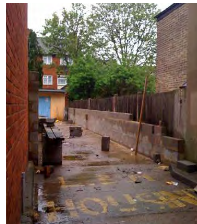
15. Photo of concrete wall being built by previous owner
