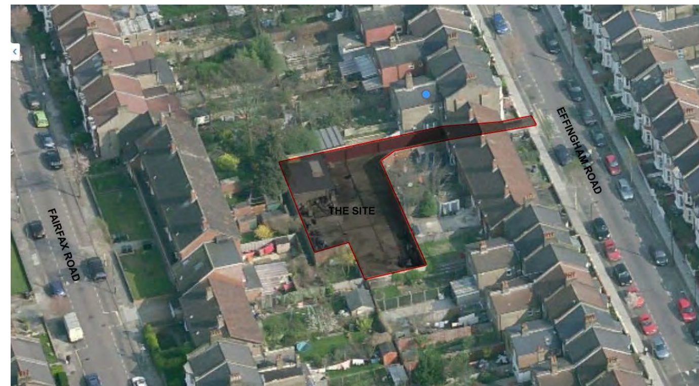
05. Aerial Photo of Site- East View
