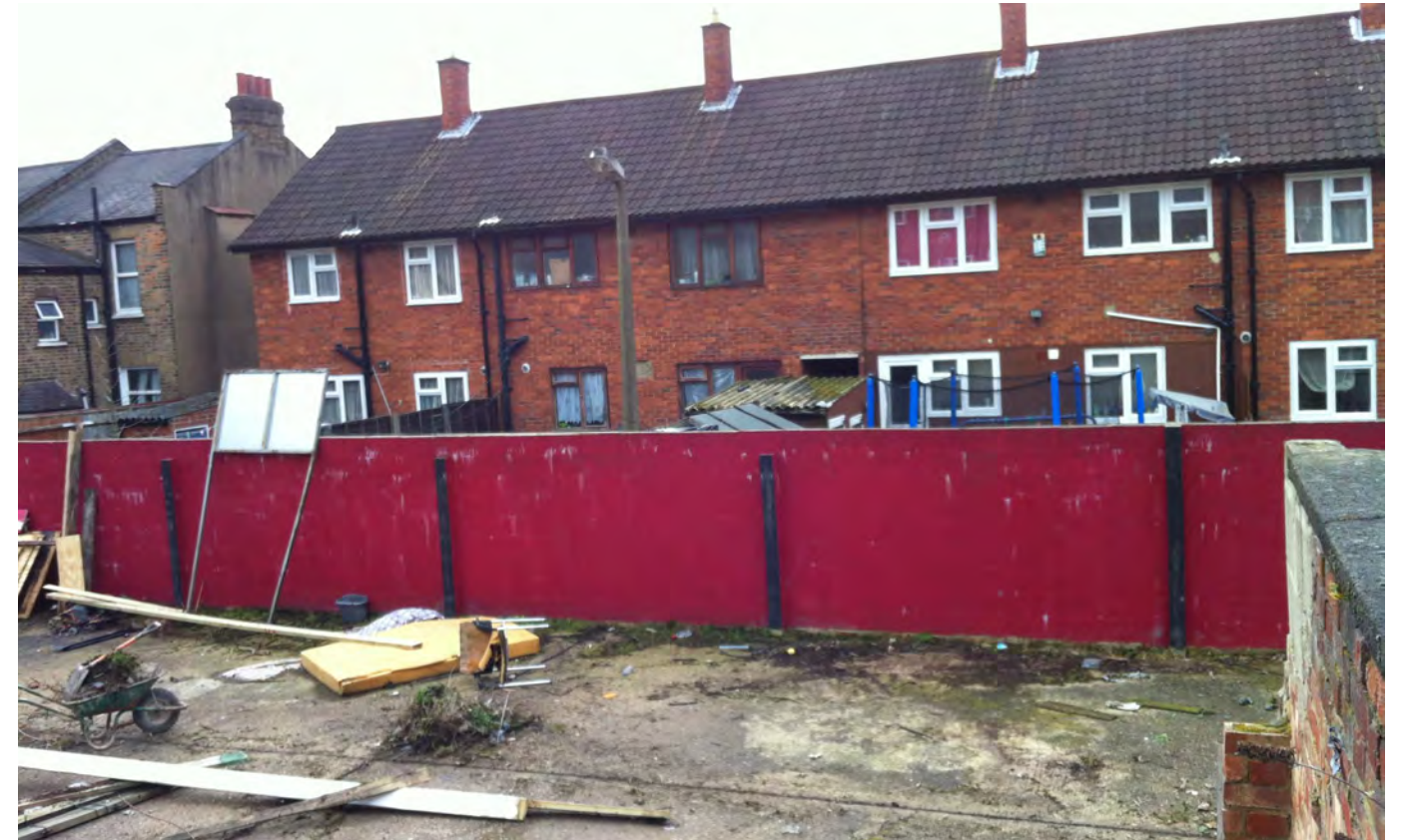
23. Photo 5 - View of site boundary wall and rear of council houses on Effingham Road
