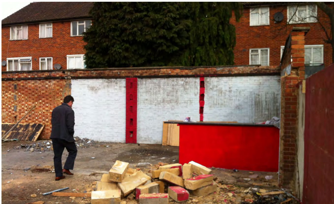
22. Photo 4 - North West view of site, showing existing boundary wall and demolition of existing shed
