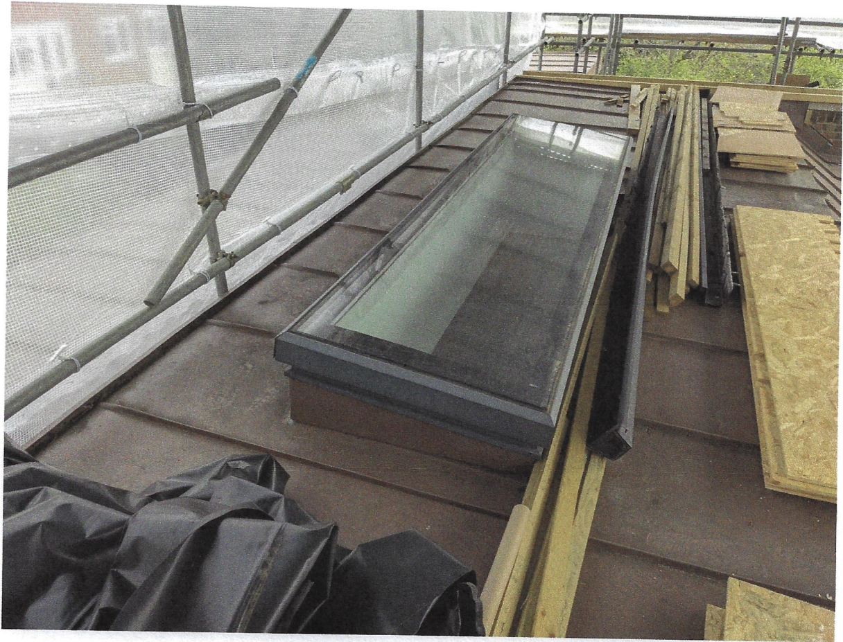
Flat Roof to Property 2
