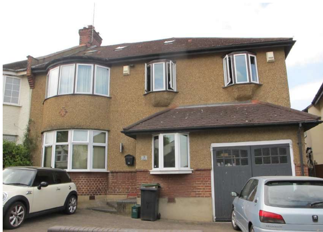
Front of Property
