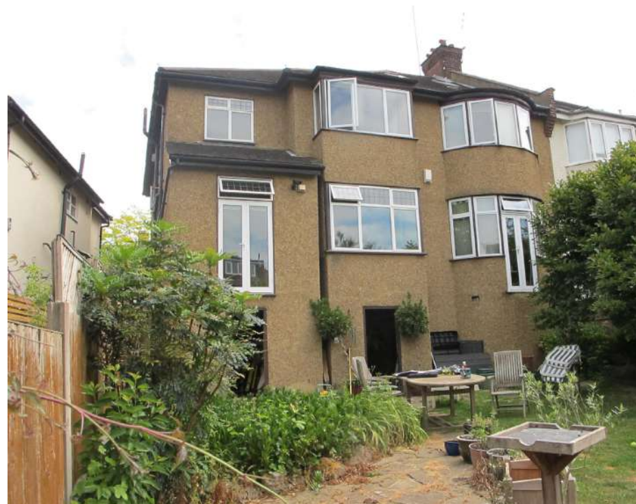
Photograph of rear of application property
