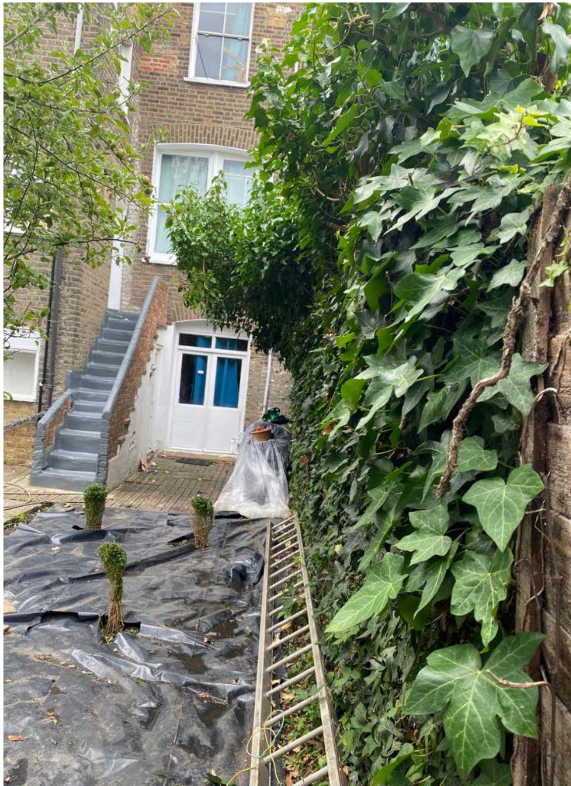
Rear of 46 Endymion Road showing boundary wall
