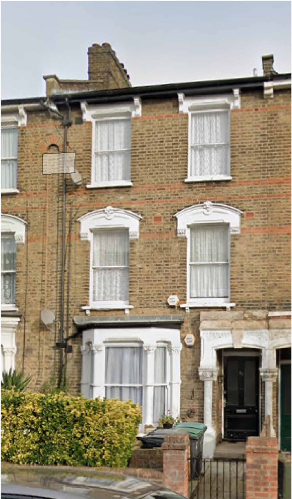
FRONT ELEVATION PHOTOGRAPH
