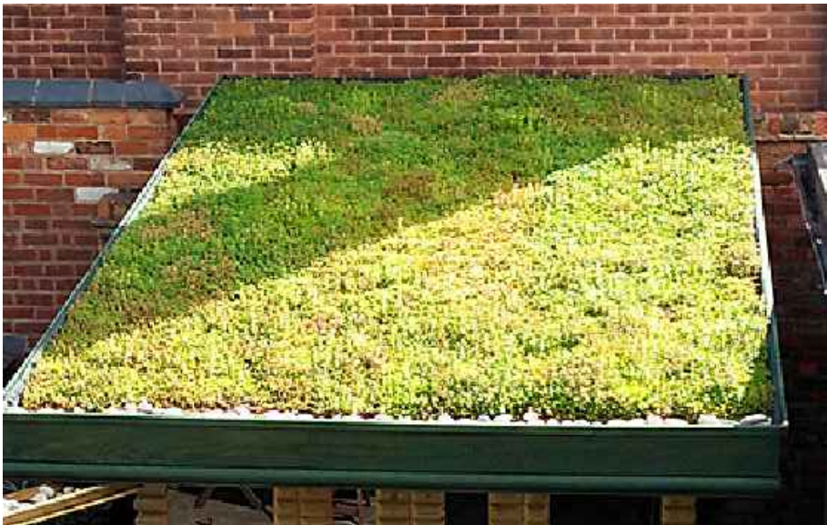
LIGHTWEIGHT GREEN ROOF SYSTEM
