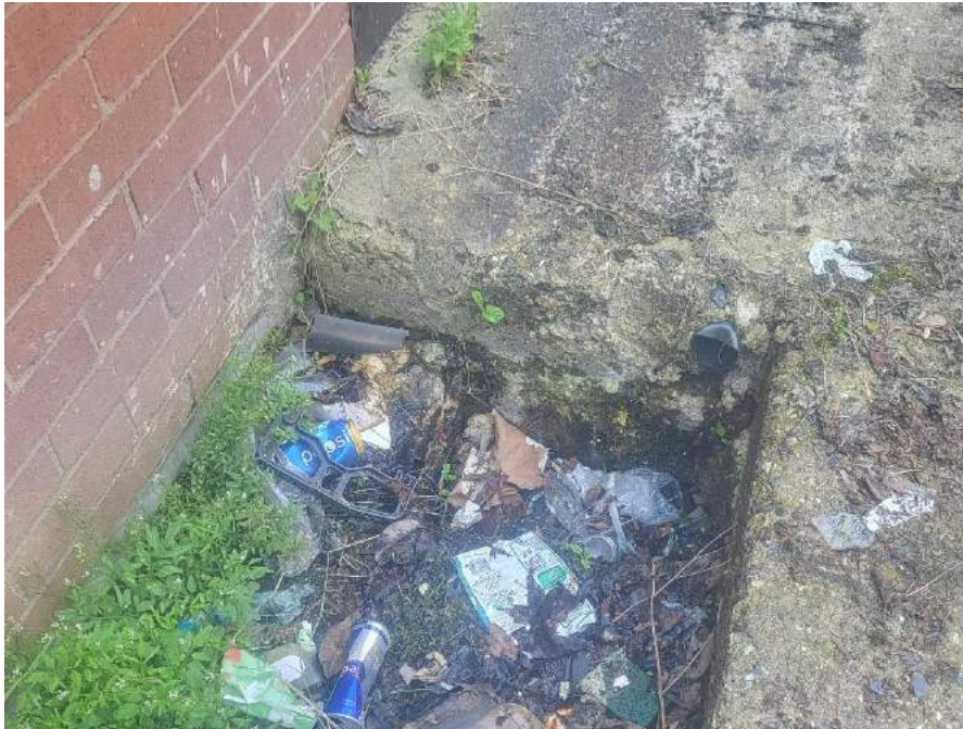
Photo 4– Drain at the rear of the site.
