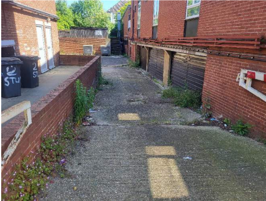
Photo 3– Rear hard standing area (facing southeast)
