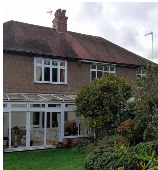
10.1 Photo showing variegated holly tree (T1) adjacent to the existing conservatory.
