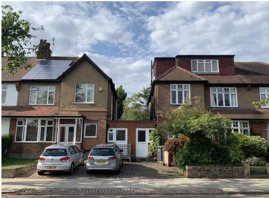
2.3 Photo showing gap between the upper floor of 49 and 51 Fordington Road. The gap measures around 3.9m at the front of the houses. The space between the first floor of buildings varies along the street from between 1 and 6m.
