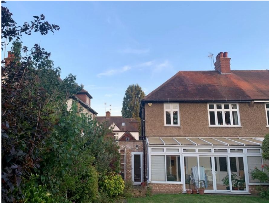
2.4 Rear of 57 Fordington Road as existing, showing disparate elements of conservatory, side extension and garage.
