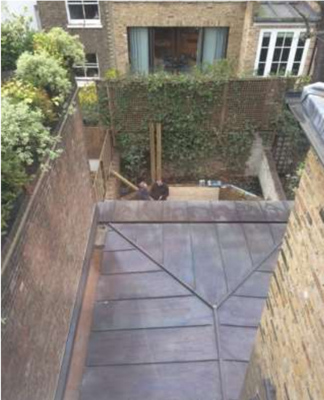
Example of a well detailed hipped metal roof by Patalab Architects (2018), copper, installed on and extension to a Grade II listed building in Westminster.
