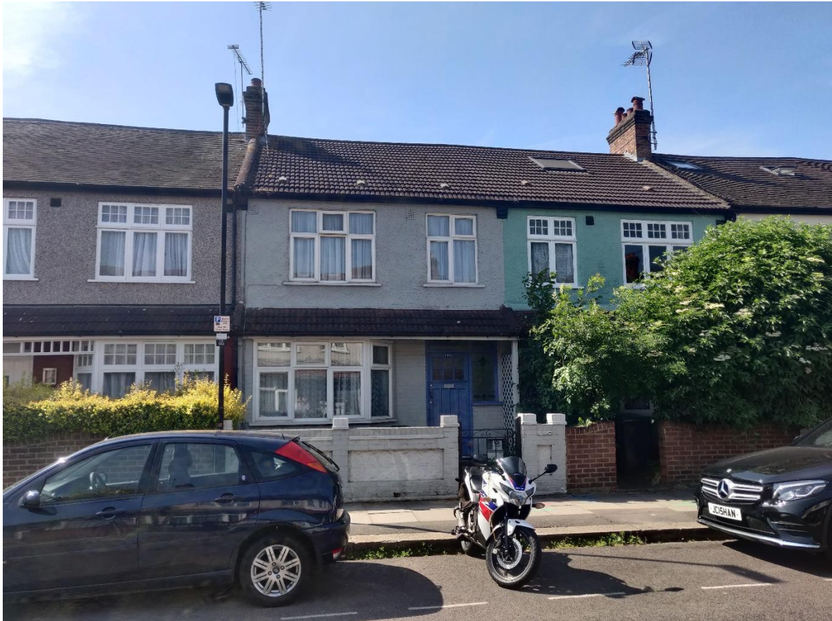
Front Elevation of no.102
