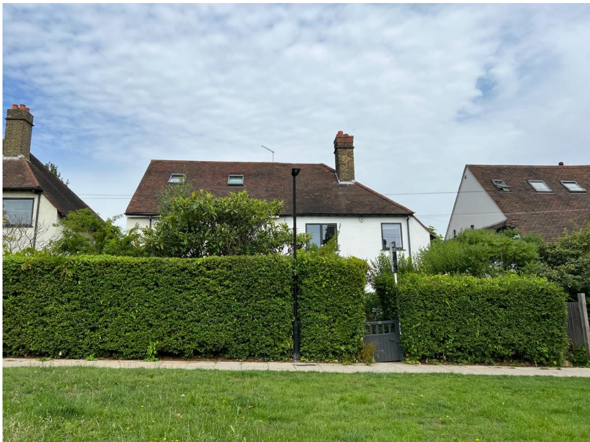
Figure 6 View of 158 Woodfield Way from Durnsford Road, Location 1
