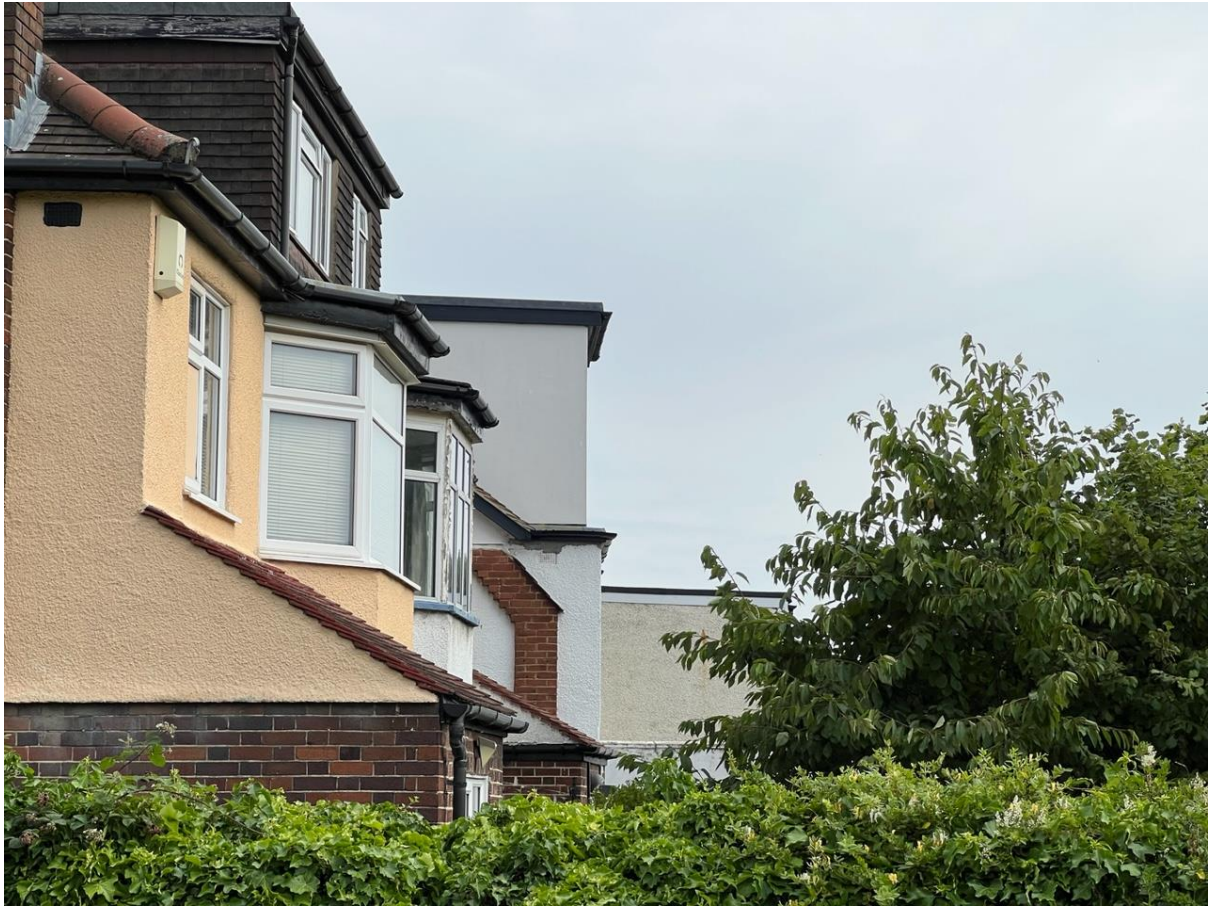
Figure 4 Photo of 15 Gordon Road with loft extending over bay window
