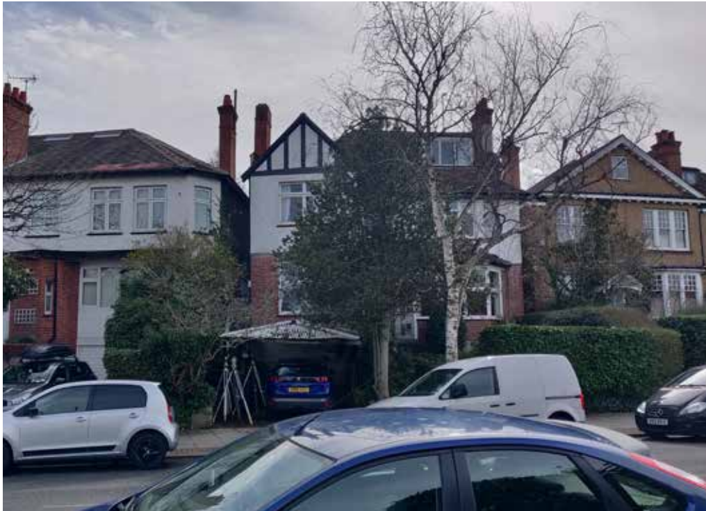
[Fig. 02] View of street facing facade of 23 Creighton Avenue.
