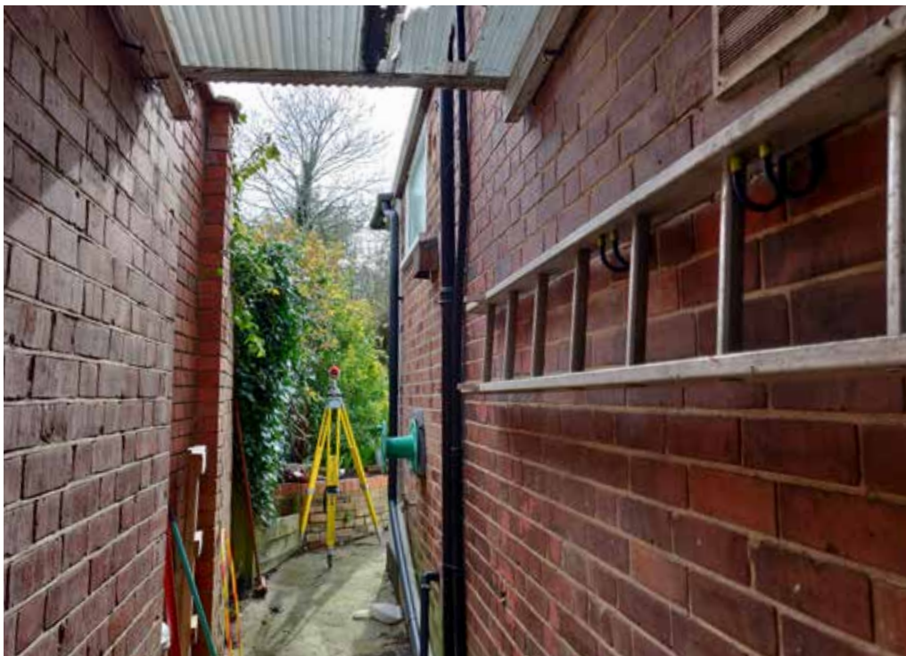
[Fig. 03] View from side alley through to rear garden.
