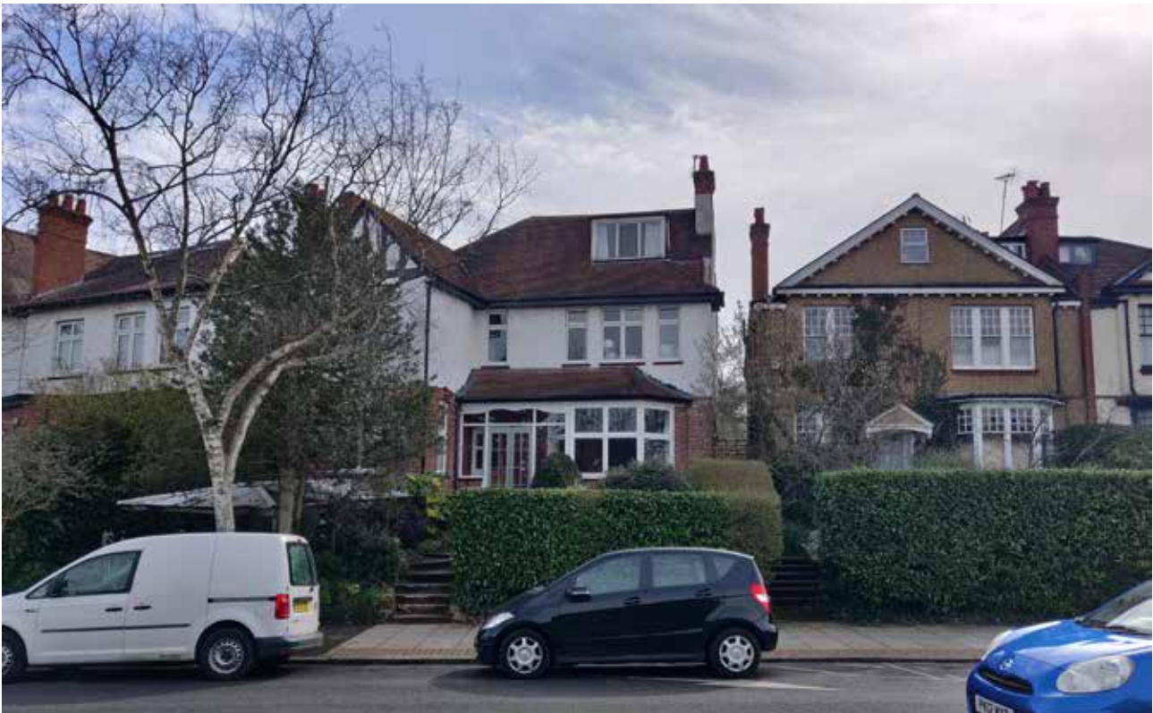
[Fig. 01] View of street facing facade of 23 Creighton Avenue.
