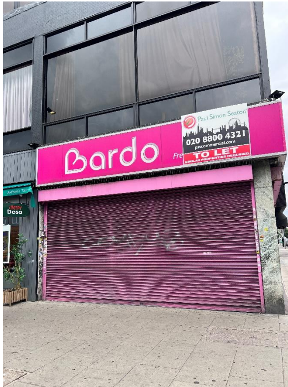
Existing South-West (front) elevation situated on the High Road
