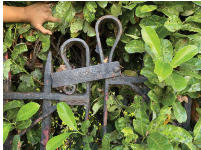
PHOTO OF 16 BRUCE GROVE RAILING DETAIL (HIGHLIGHTING FINIAL)
