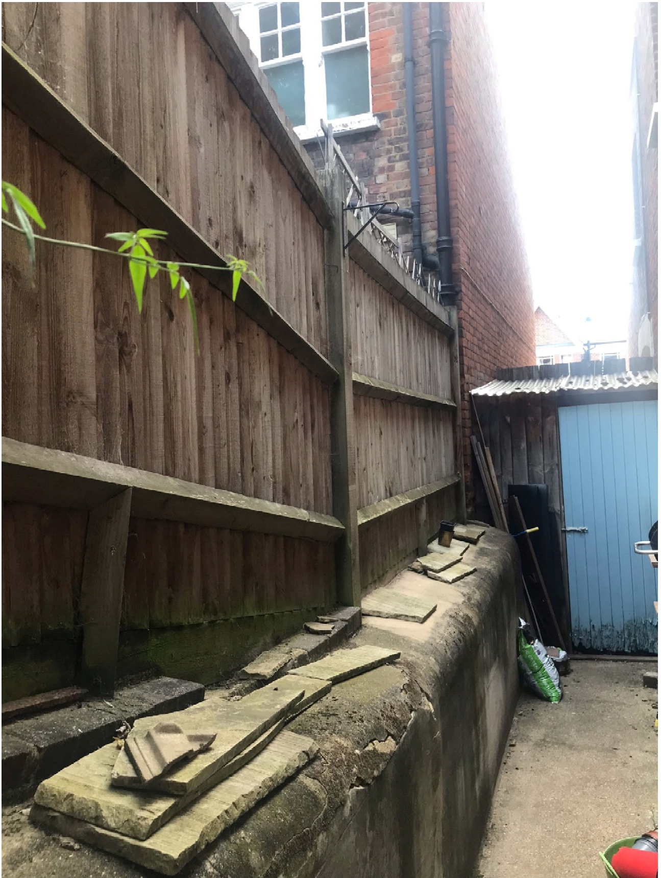
Side passage of No 30 showing 1 metre high retaining wall (passage is approx. 1 metre below floor level of No 32)
