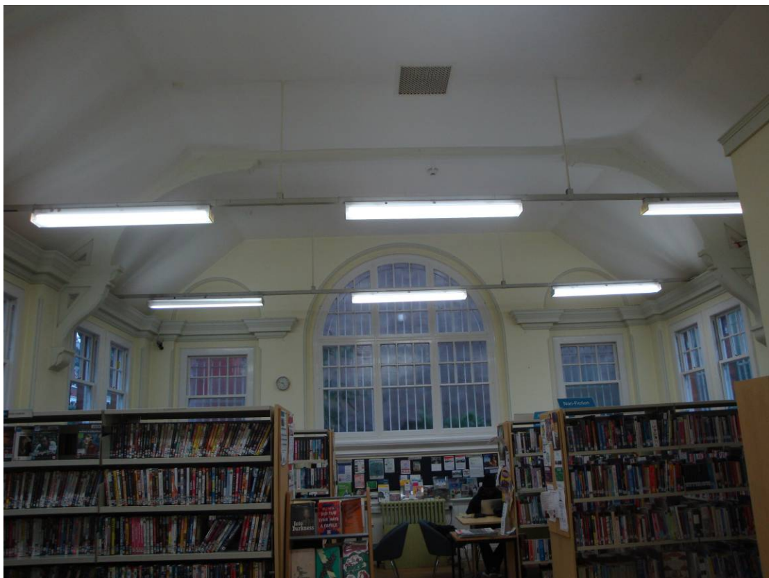
Stroud Green Reading Room for comparison ( 1901) Stroud Green Library Reading Room roof (1901). Note generous daylight on three sides
