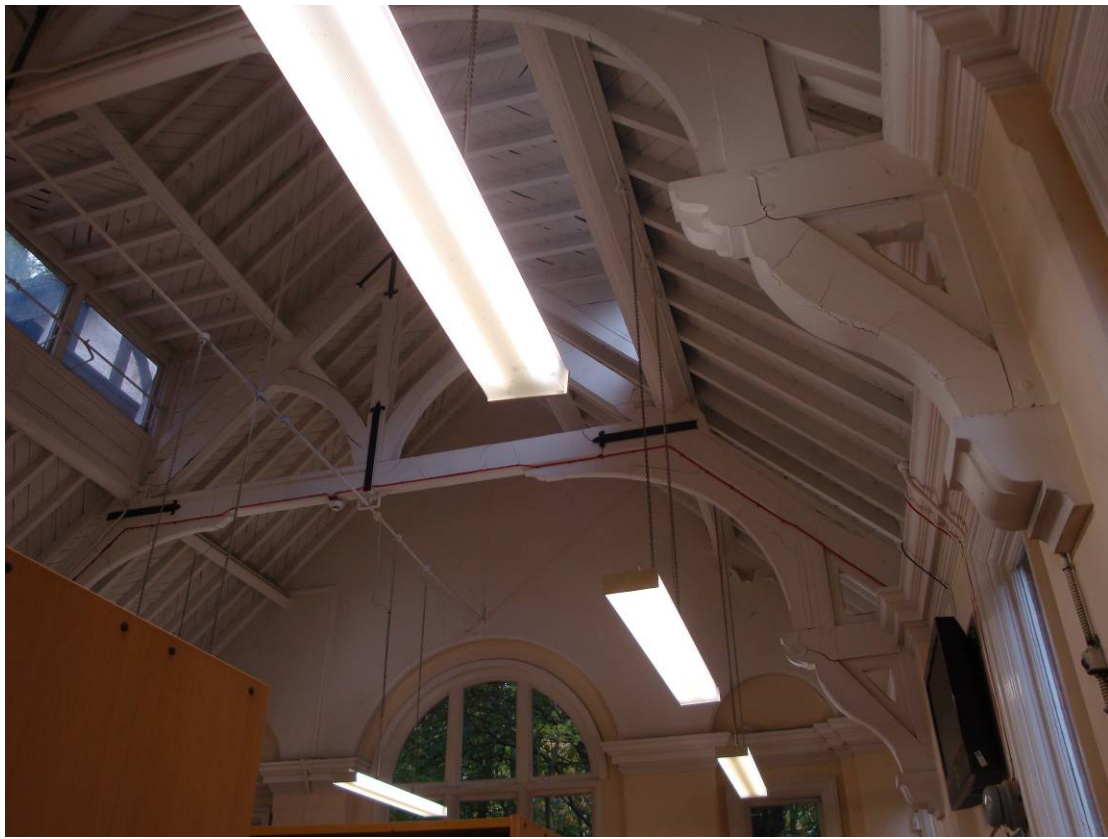
Highgate Library Reading Room roof (1902). Daylight available on only two sides so clerestory windows used on the long sides
