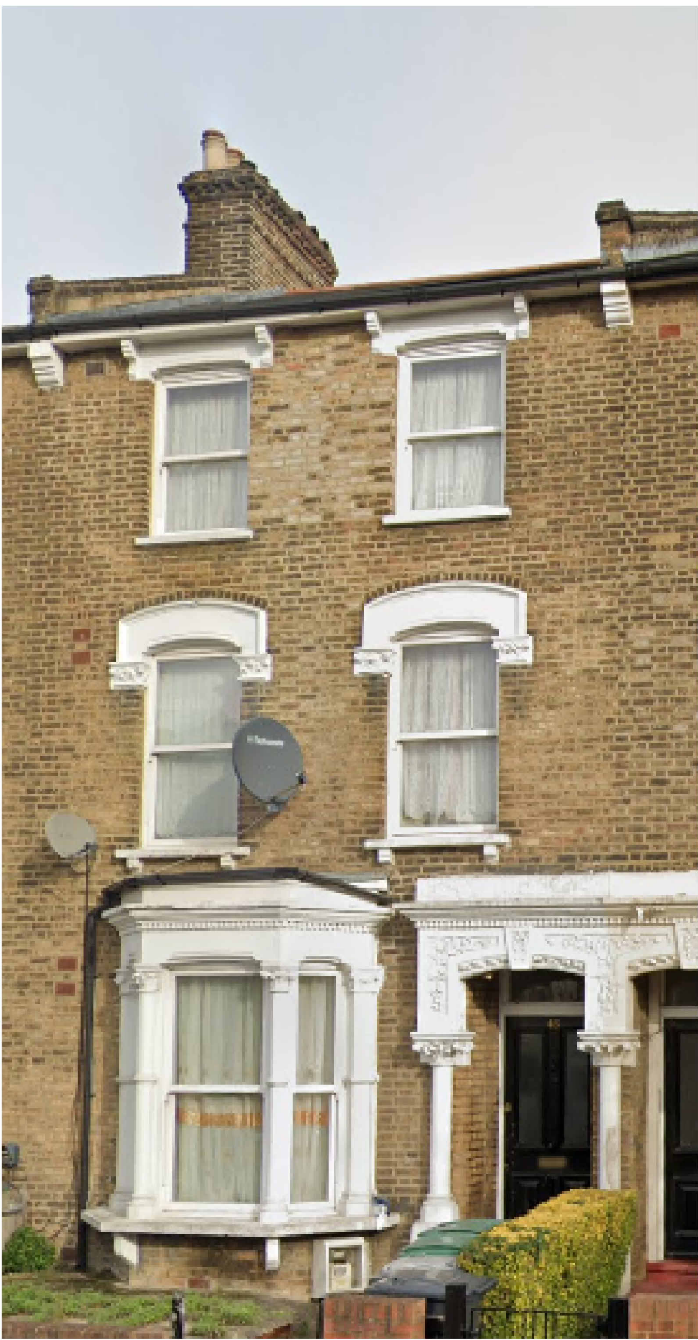
FRONT ELEVATION PHOTOGRAPH
