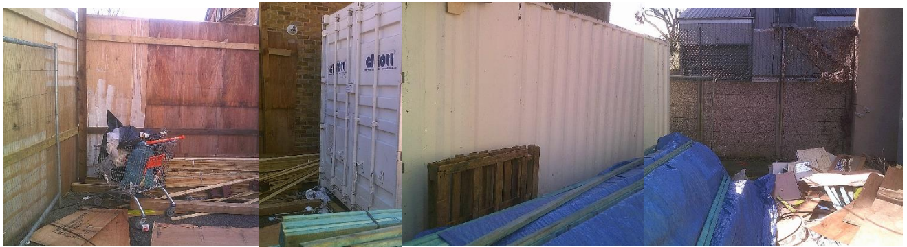
Internal view of the site towards south-west.
