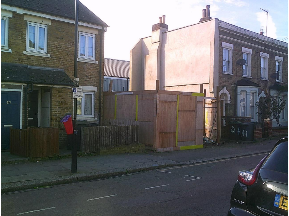
Photograph 1: View of the site, view from Antill Road towards west.
