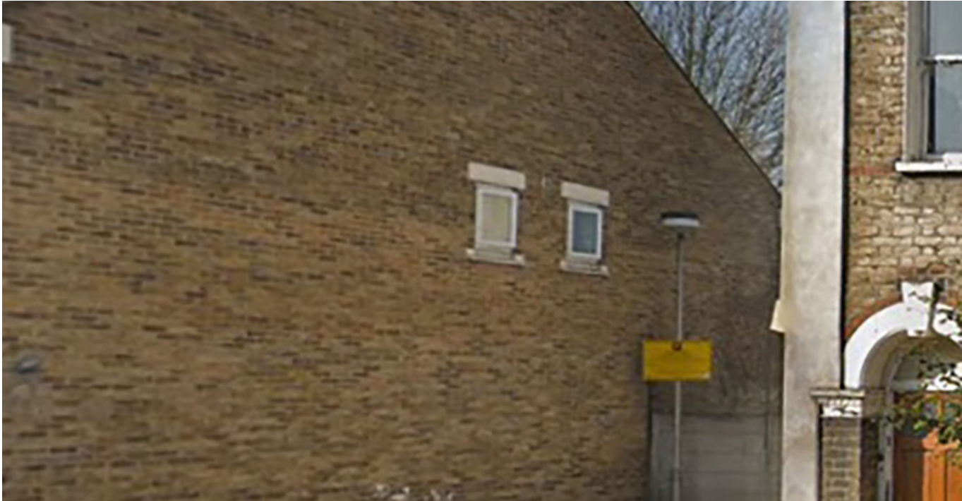
4.2 View of the windows in the flank wall to 39 Antill Road
