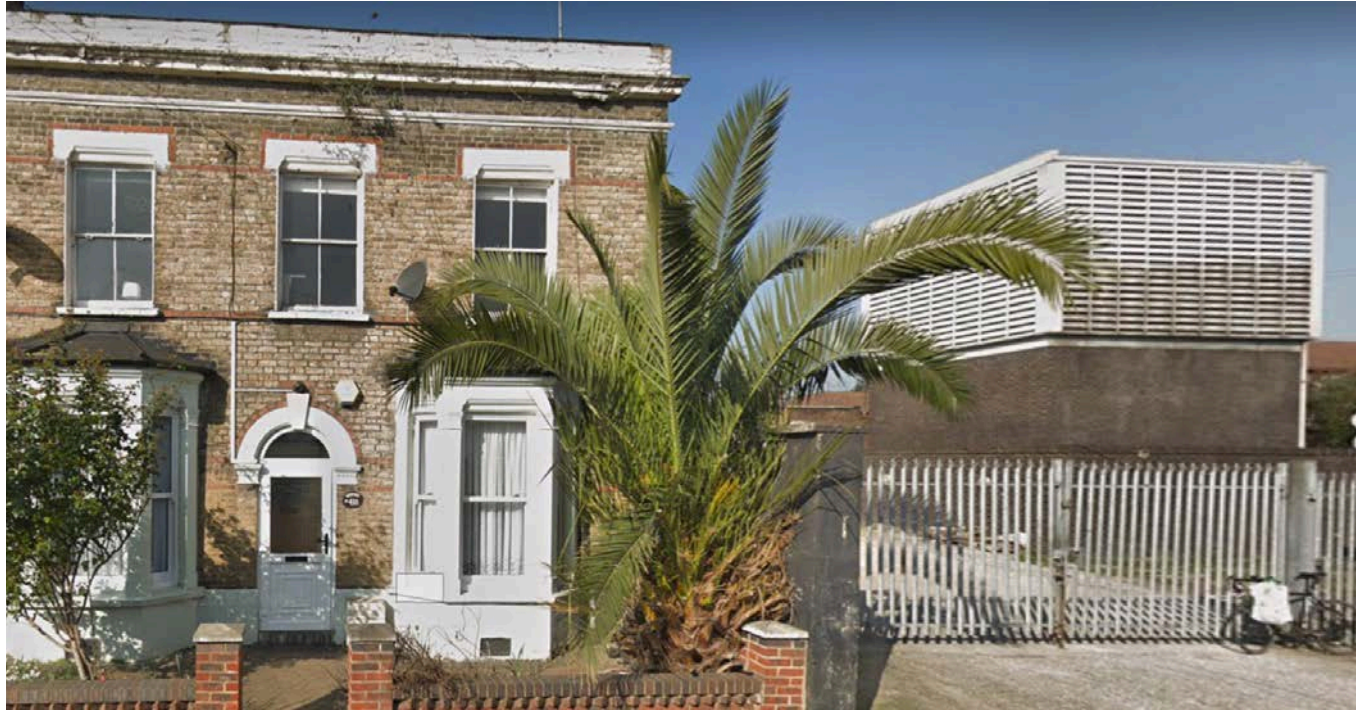
4.5 View of the TfL infrastructure adjacent to 41 & 41a Antill Road
