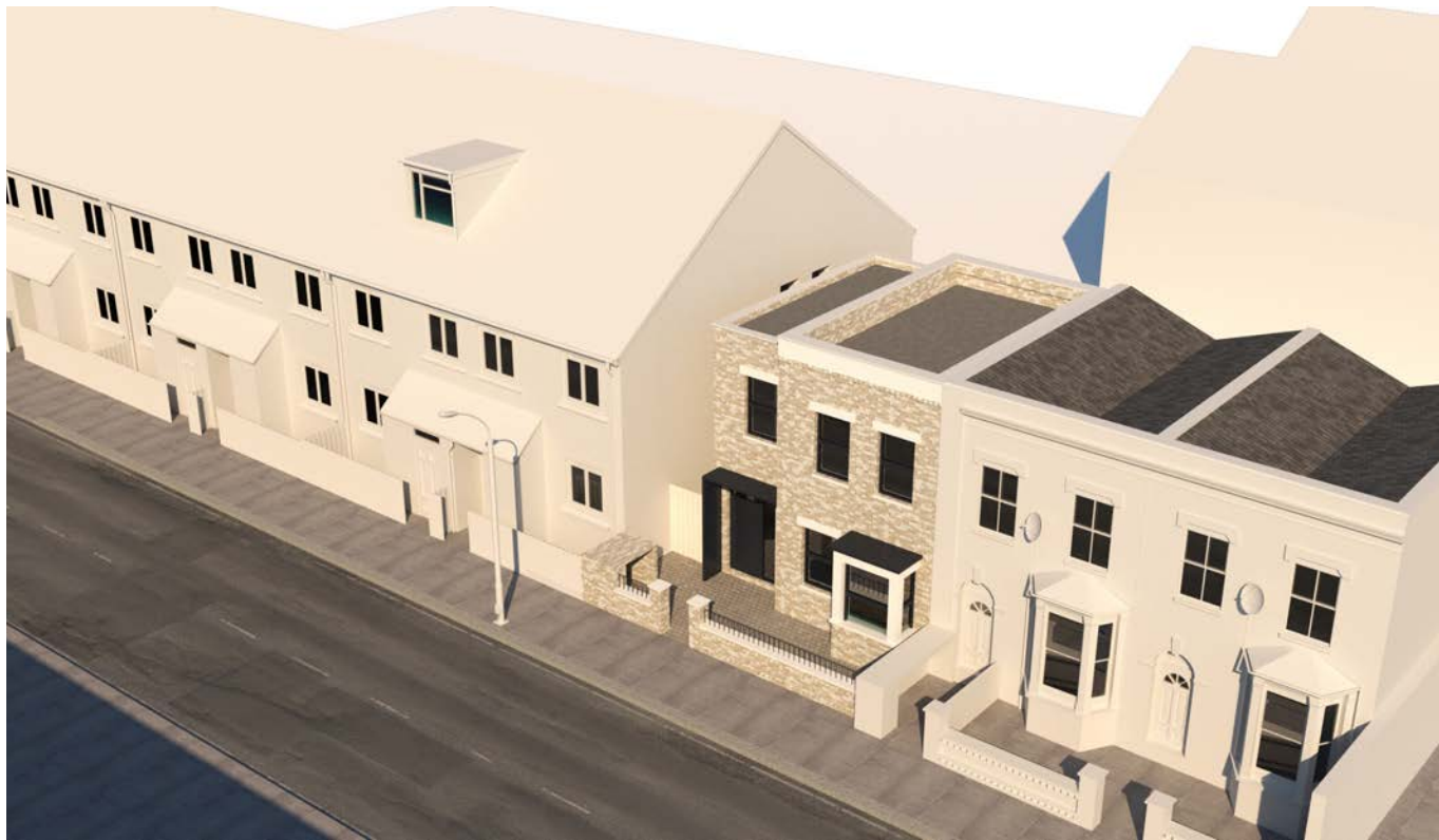
14.3 Aerial view of the proposed house
