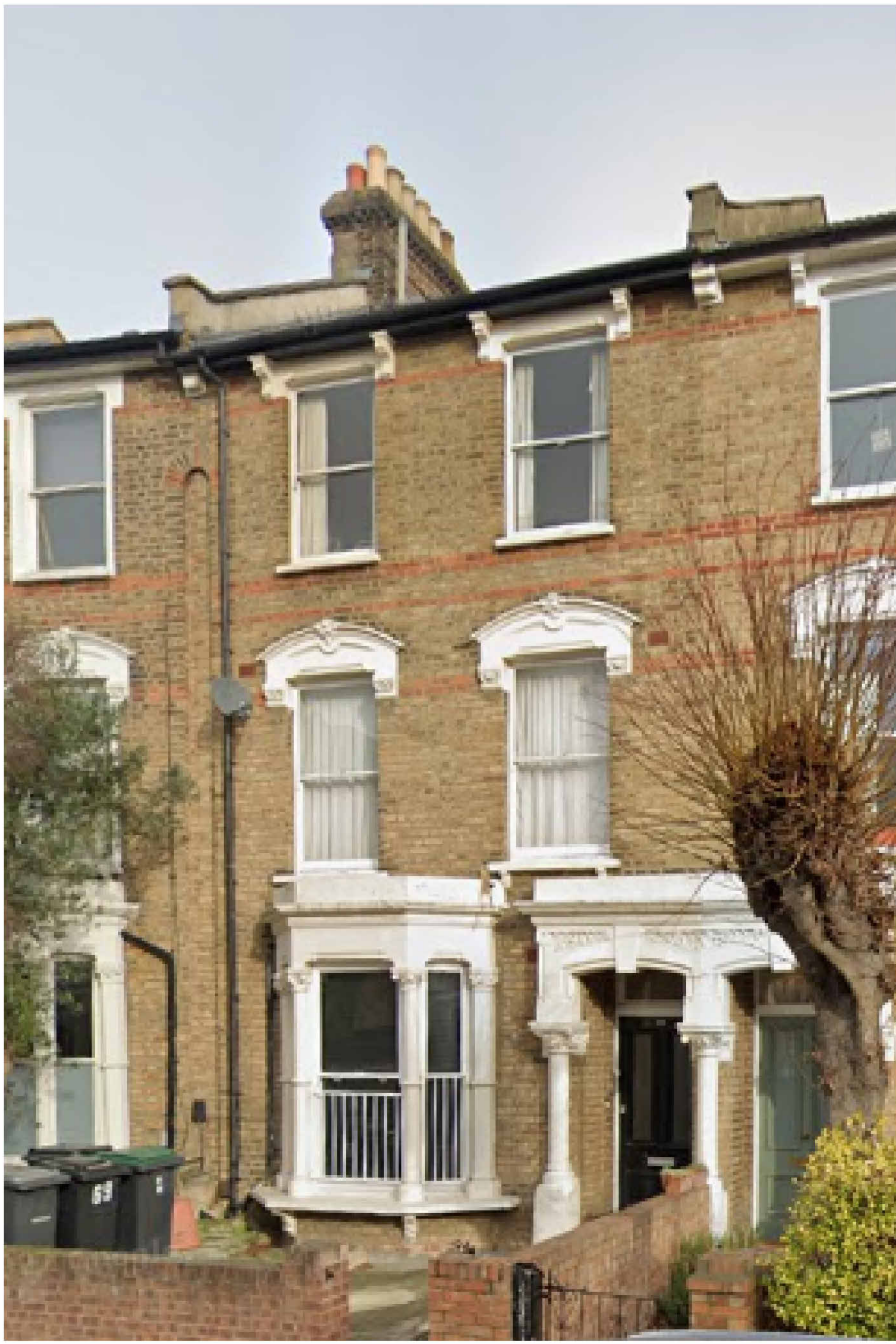
FRONT ELEVATION PHOTOGRAPH
