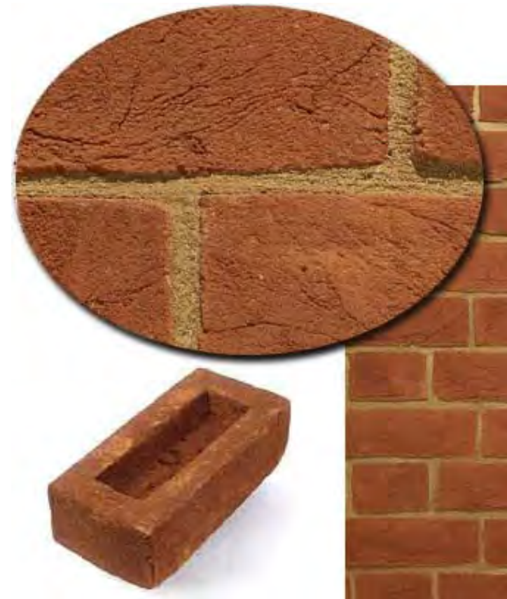
1. Lambs 'red rubber' brickwork to match existing
