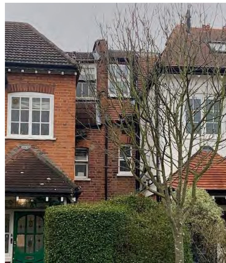
5. Similar roof infill on Leaside Avenue
