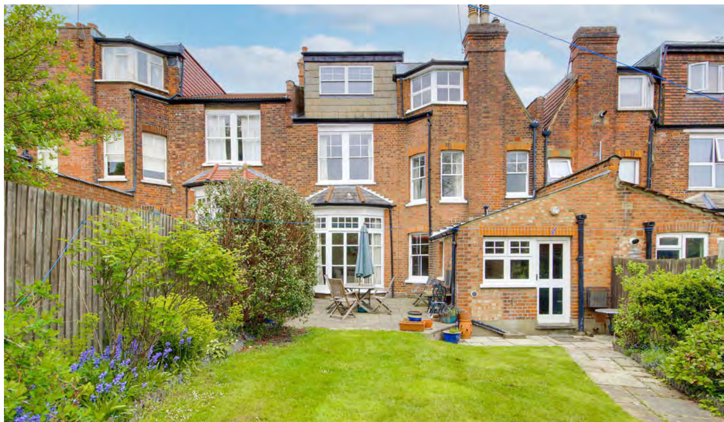
4. Existing rear elevation viewed from garden
