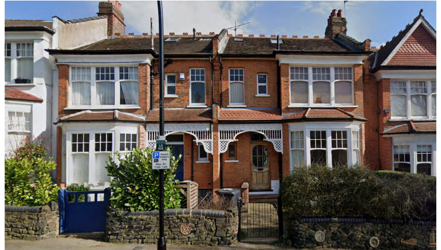
1. Precedent - Properties directly opposite at 44 & 46 Leaside Avenue with brickwork to ground and first floors
