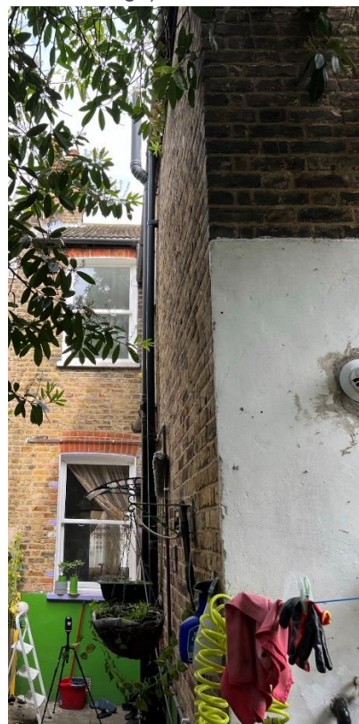
Rear elevation Windows
