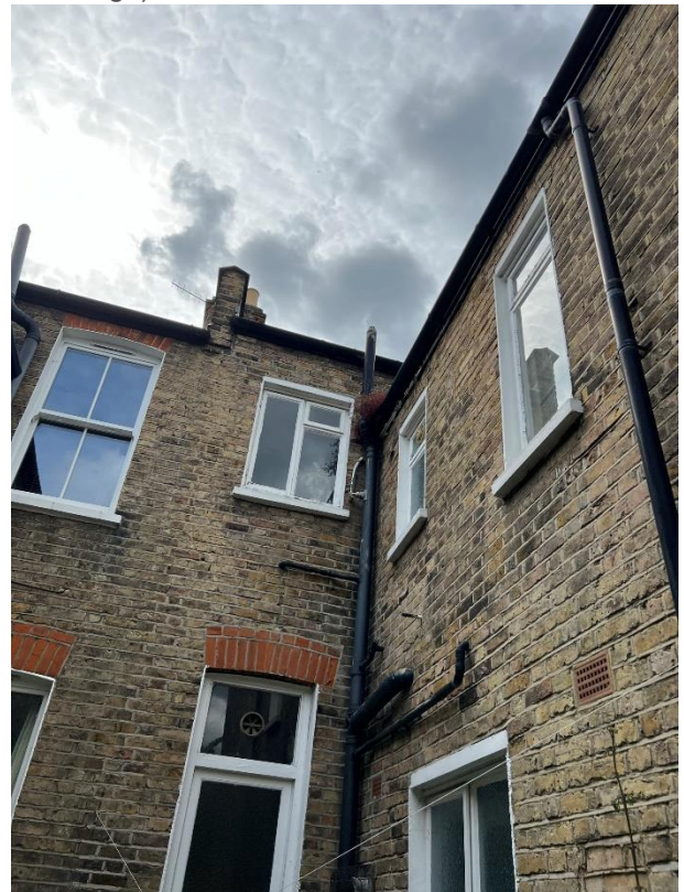
Rear elevation Windows
