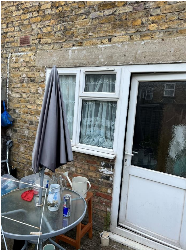
Rear exit door 2
