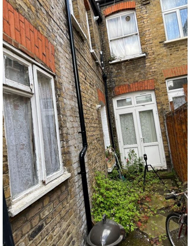
Rear exit door 1
