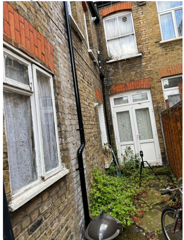
Rear elevation Windows
