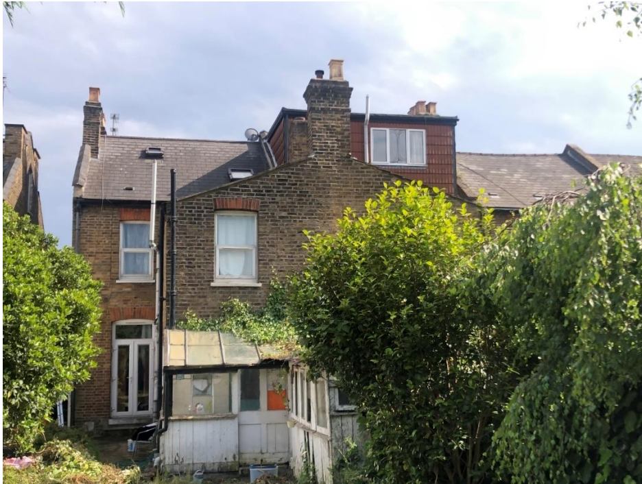
Rear view prior to construction of loft.
