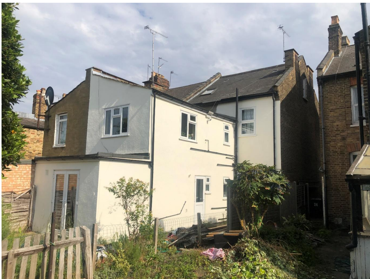
The rear outriggers are well set back from the site boundary
