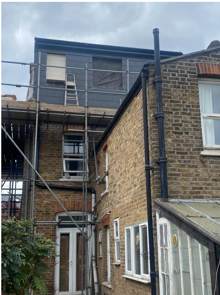
Rear view with loft dormer constructed
