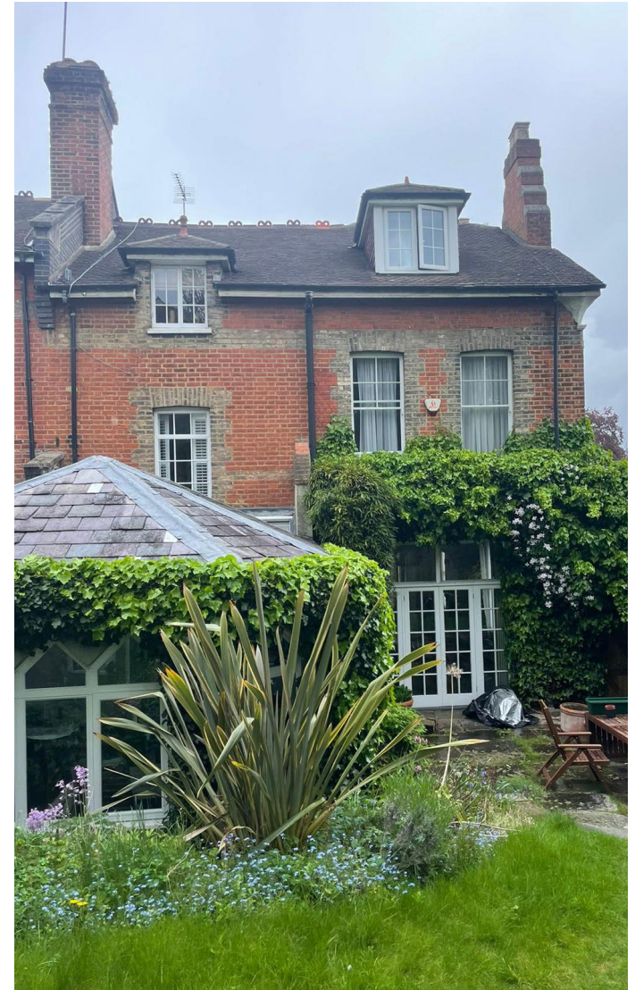
23 Wolseley Road rear garden view. The proposed terrace will replace the second floor dormer window on the top right
