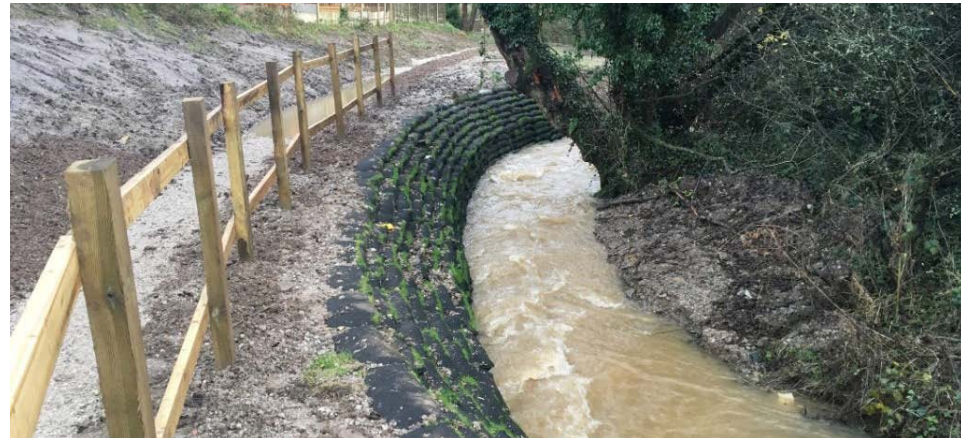
Figure 15 - Pre-establishment of inlet feature
