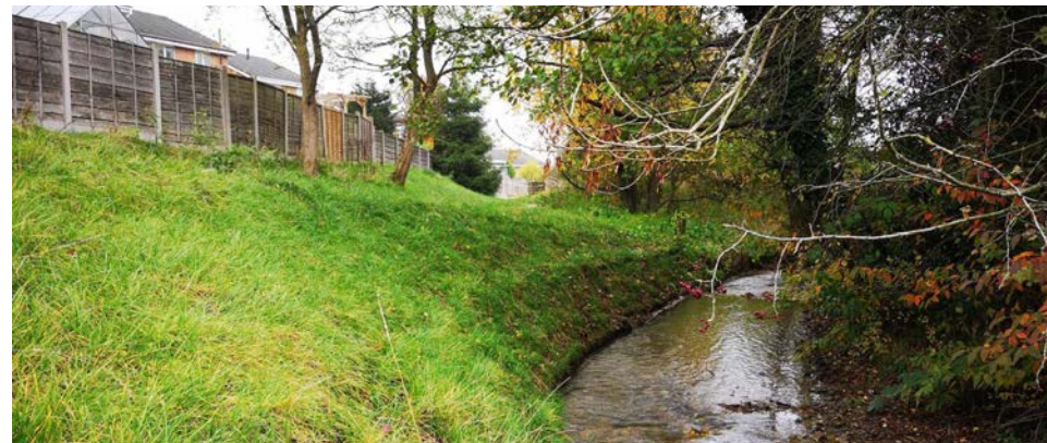
Figure 16 - Post-establishment of inlet feature
