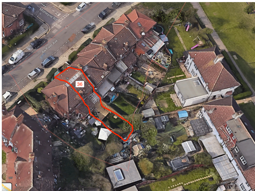
Photo of Site – (Rear Elevation) and Photo of Next Door Extension
