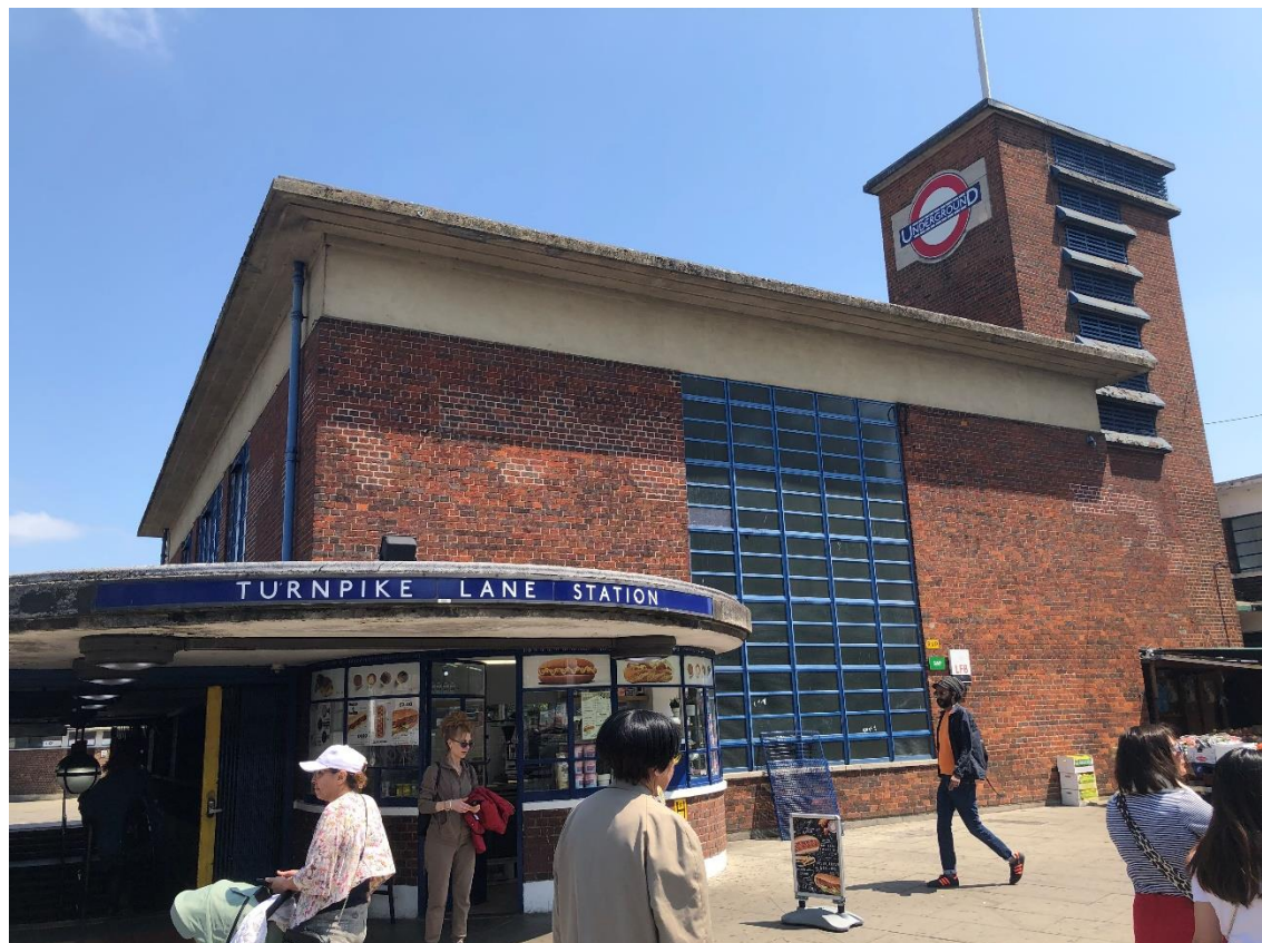
Photograph 6 Turnpike Lane Tube Station
