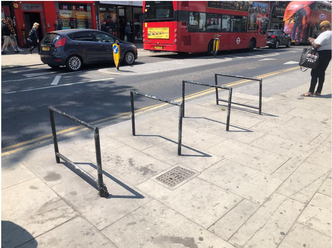
Photograph 4 Cycle Stands along the A105 High Road
