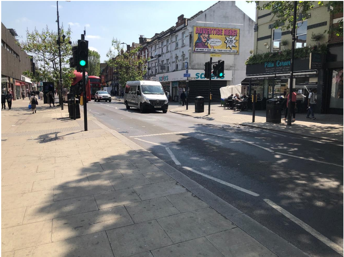
Photograph 3 Footways and Formal Pedestrian Crossing across the A105
