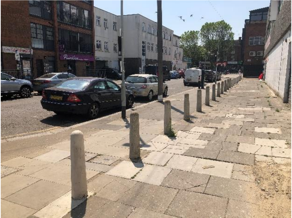
Pedestrian Footway along Whymark Avenue
