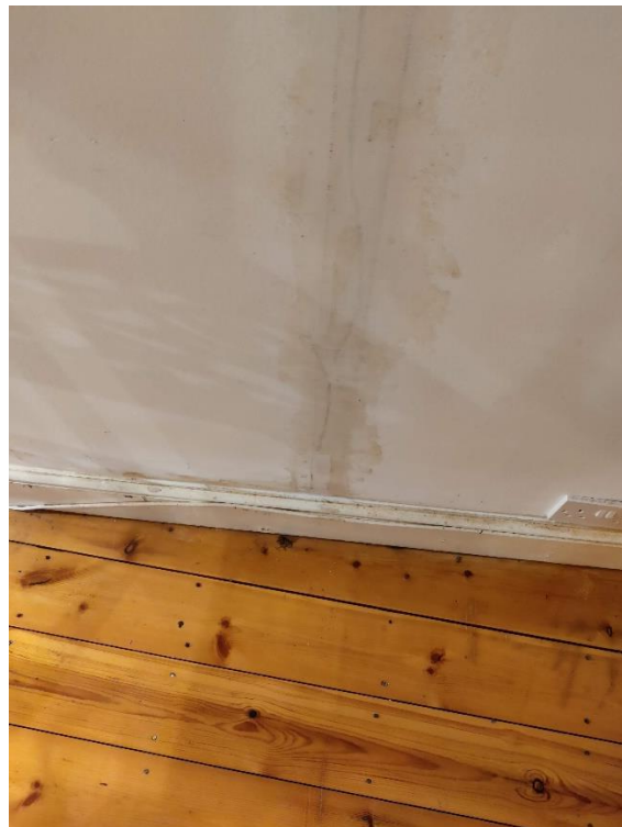
Structural cracks of more than 1cm width to side extension that have been taped over
