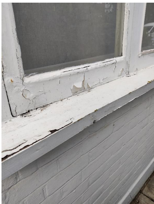
Poor condition of timber windows including rot
