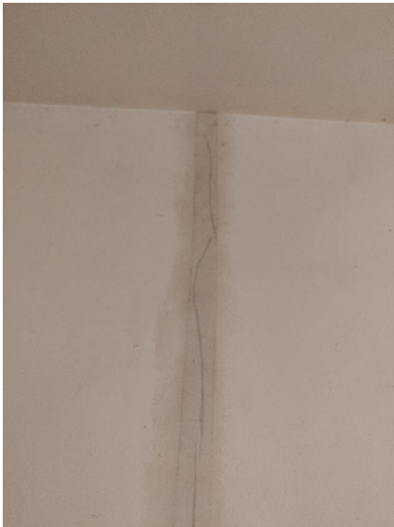
Structural cracks of more than 1cm width to side extension that have been taped over
