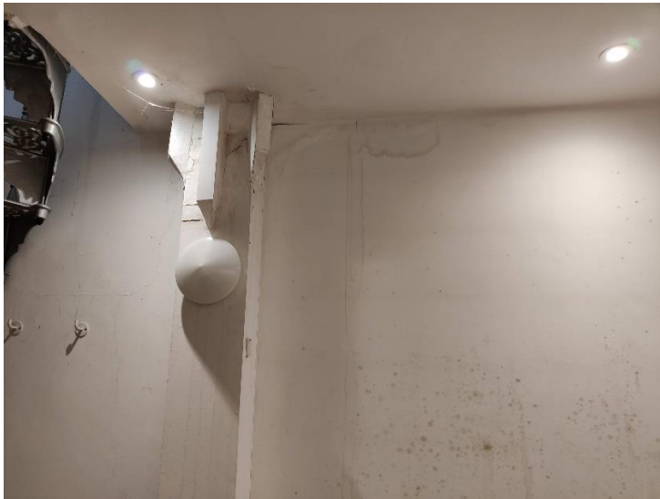
Internal damp and leaks to the external wall and ceiling
