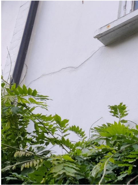
External cracks to render walls
