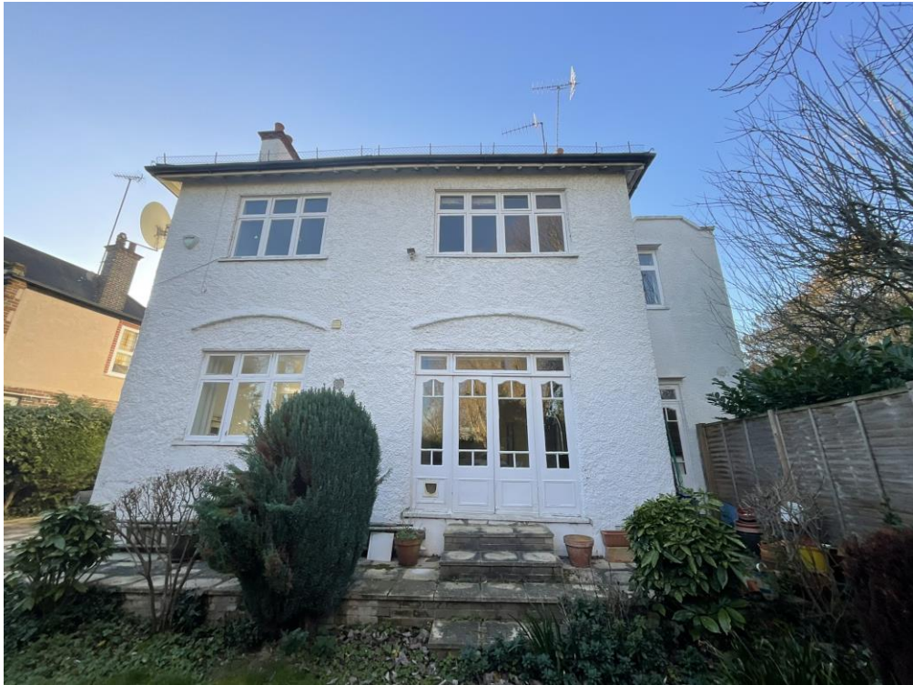
Rear elevation of the house
