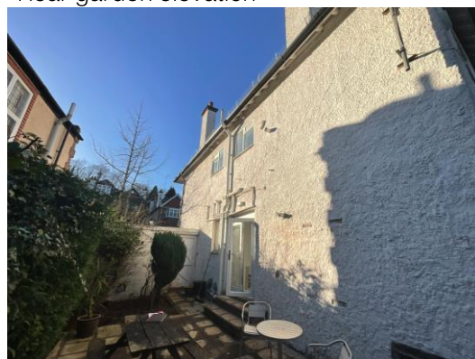
View of the south side of house
