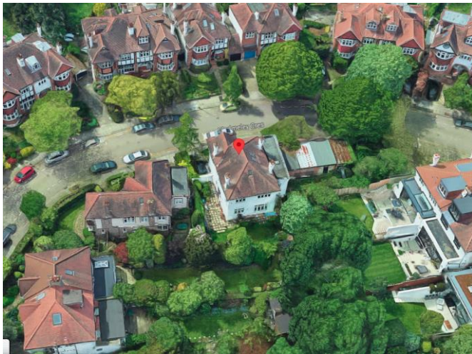
East Aerial View
