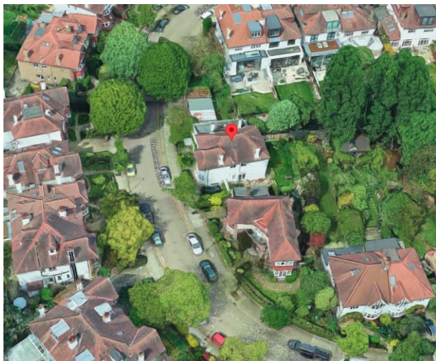
South Aerial View
