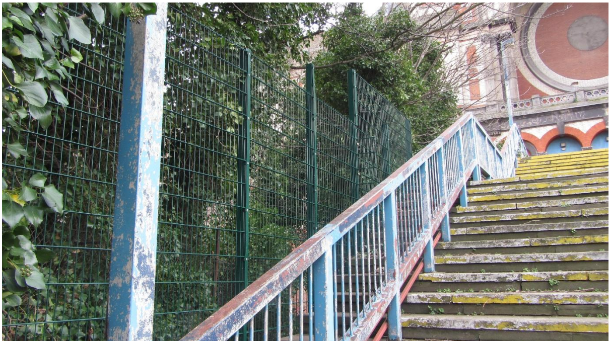
Great Hall Bridge fire escape steps/woodland and vaults under
