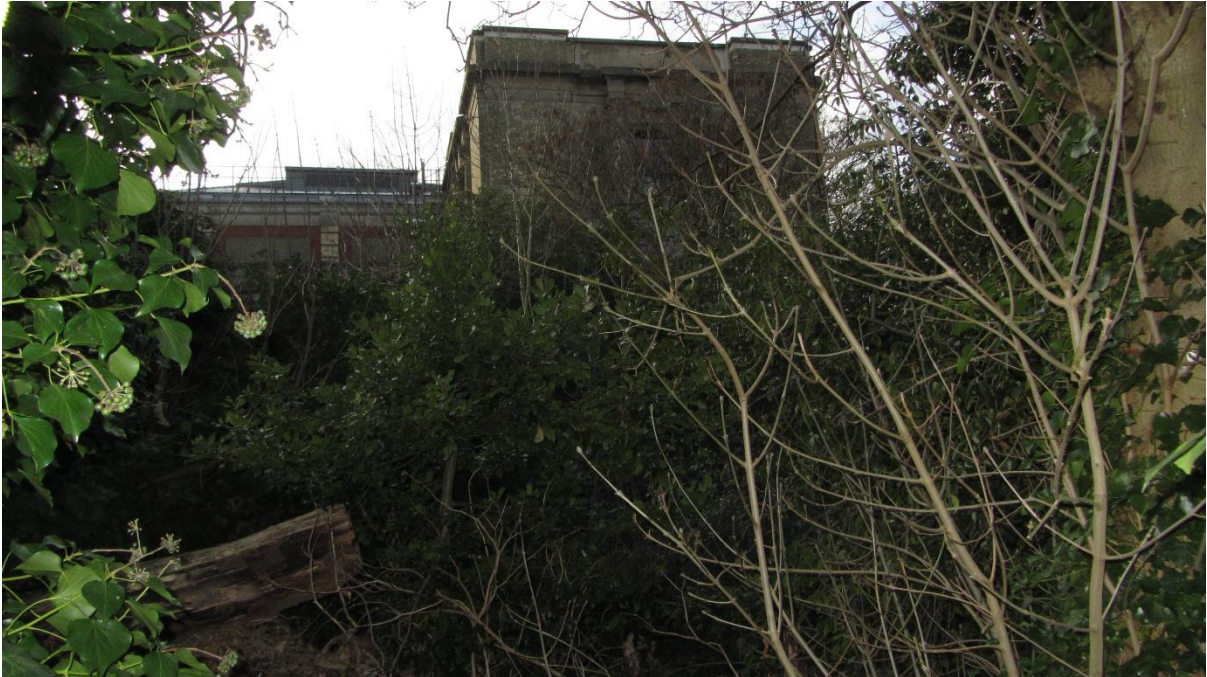
NSY/NW Tower fence (South end)
