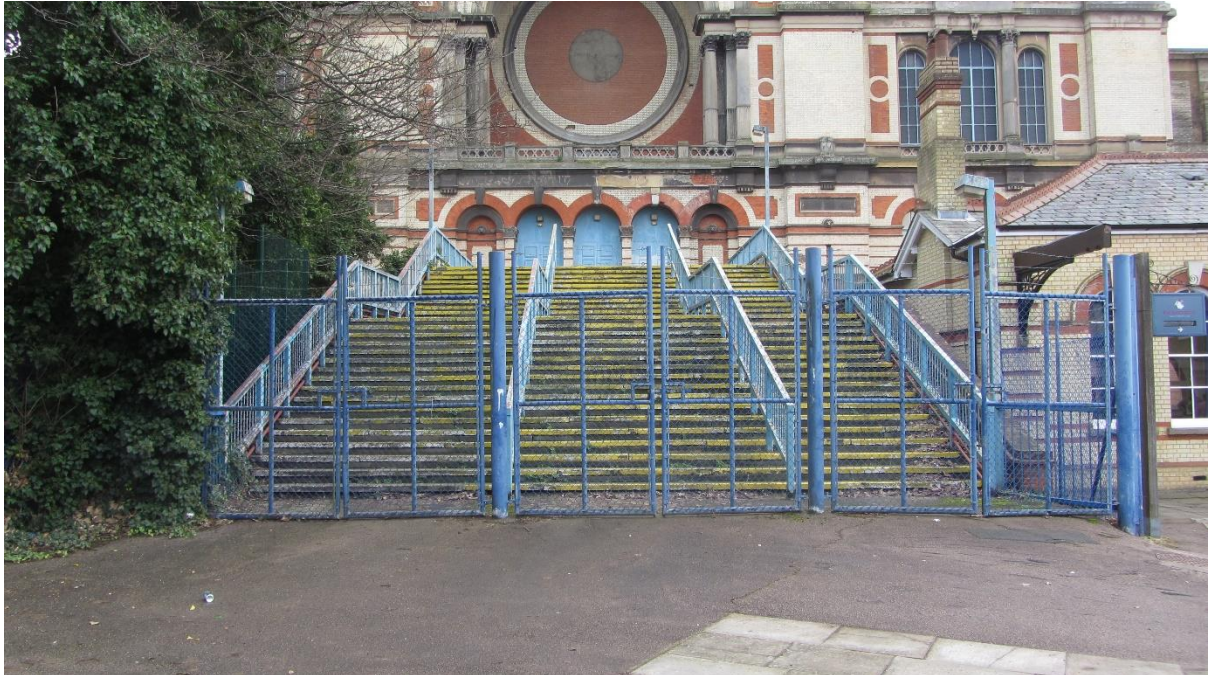
Great Hall Bridge fire escape main gates
