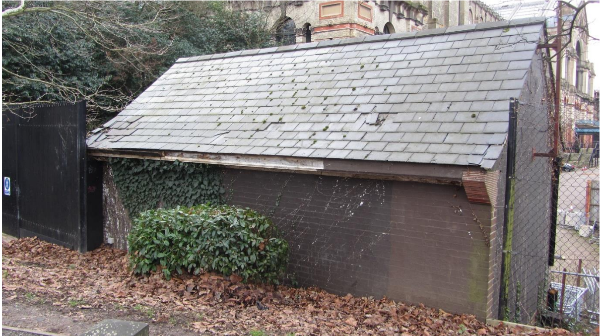
Old Paint Store
