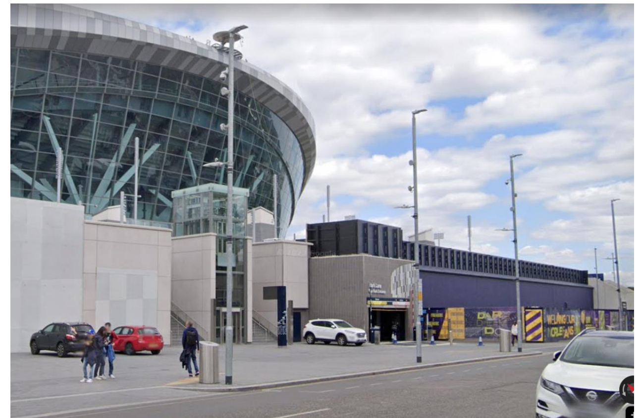
Figure 5.6 – Existing Street lighting installation along Park Lane. Image Google Maps 2023
