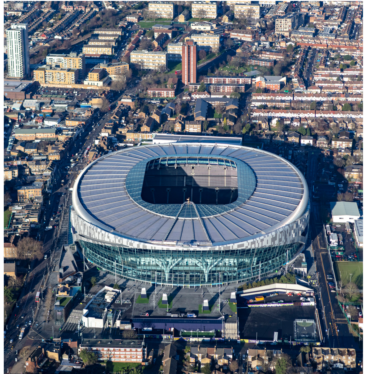
FIGURE 6. Aerial View of the Southern Development Looking North
