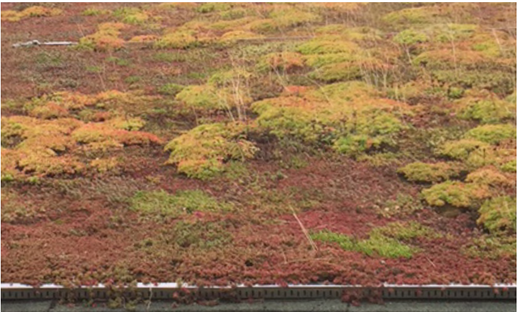
sedum roof: a low maintenance biodiverse covering that aids rainwater attenuation.
