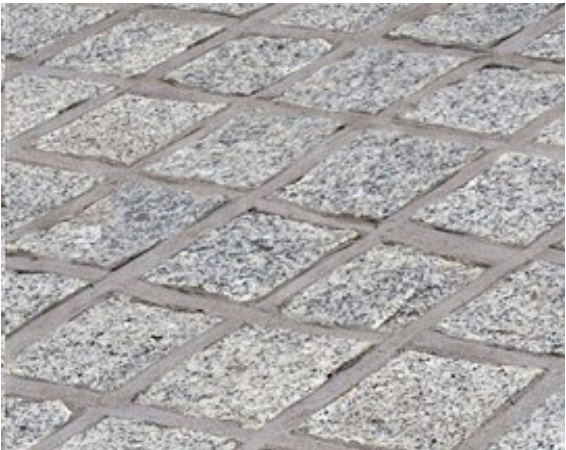
Sawn granite setts and tiger mulch surface to community garden
