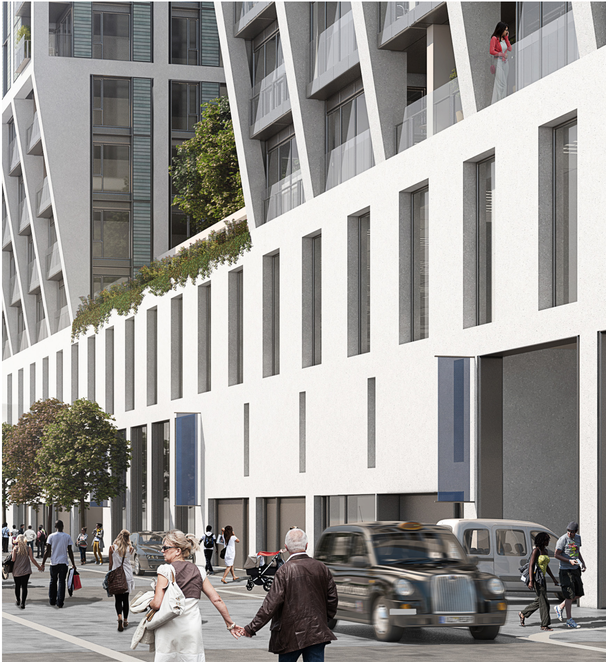
View from Worcester Avenue
