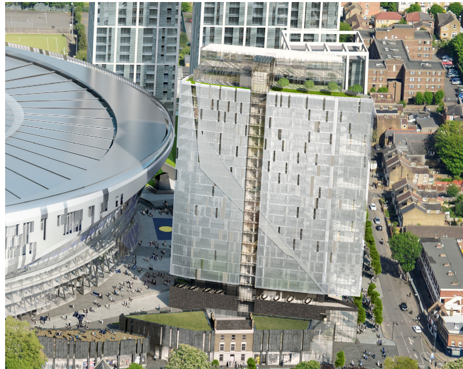
FIGURE 32. West Aerial View
