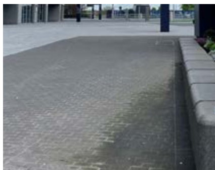
Existing paving at podium level
