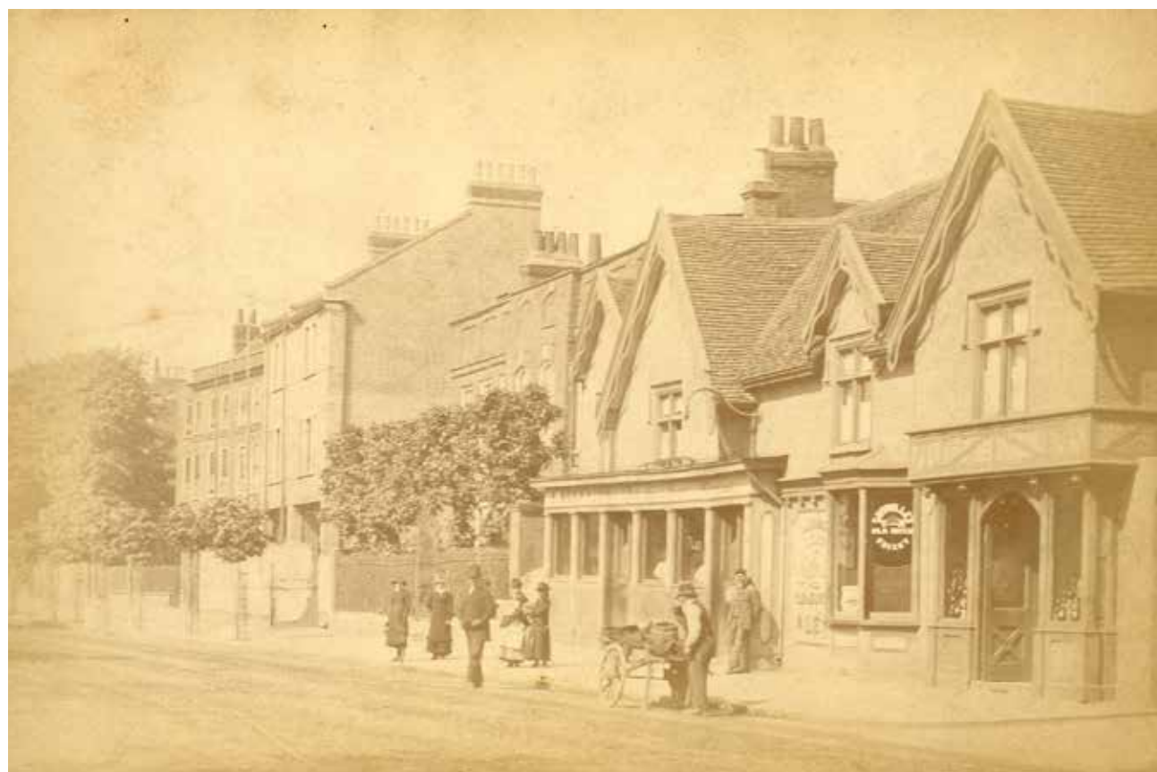
Figure 22. 750-755 High Road c1880-5
