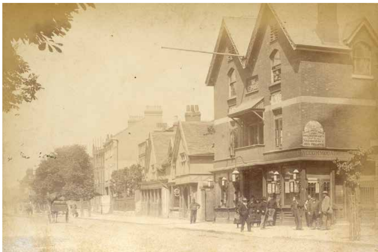
Figure 20. 748-756 High Road c1880-85
