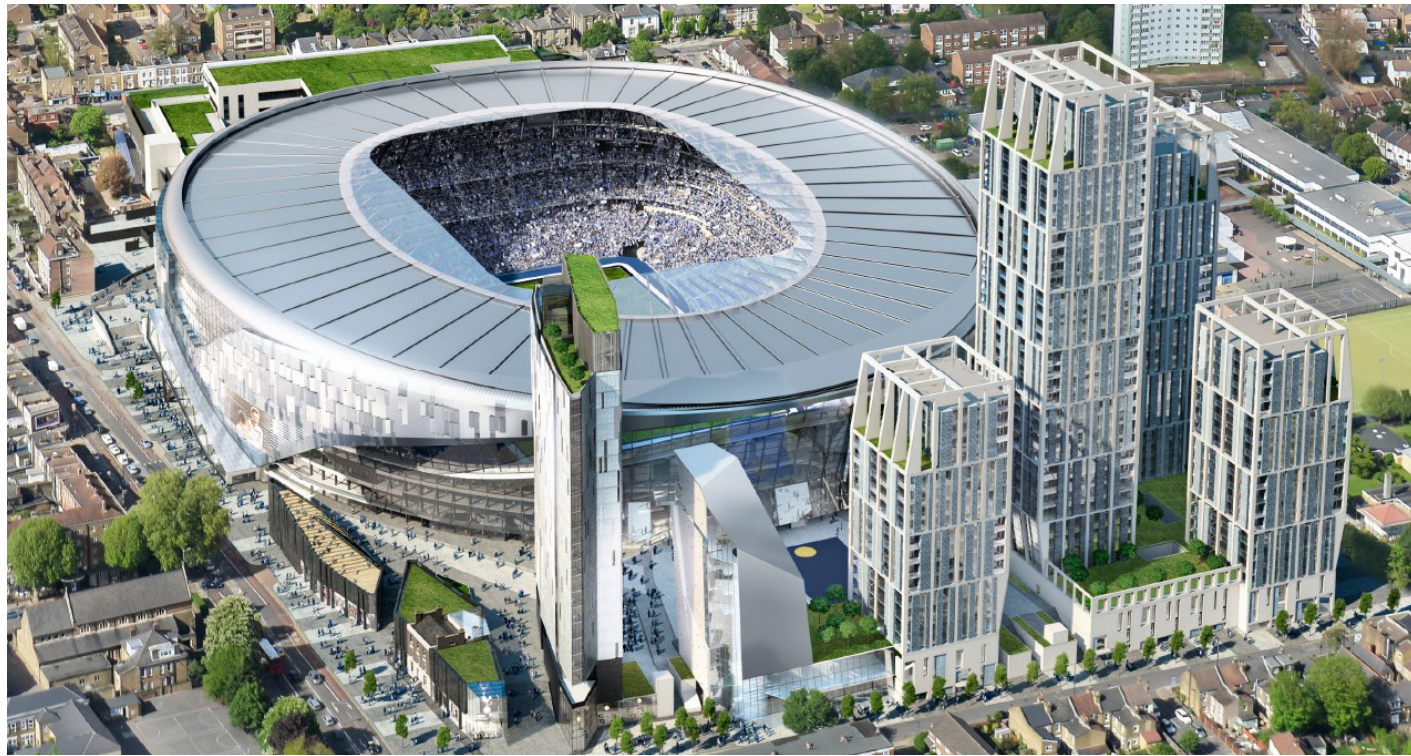
FIGURE 28. Park Lane Elevation - Aerial View
