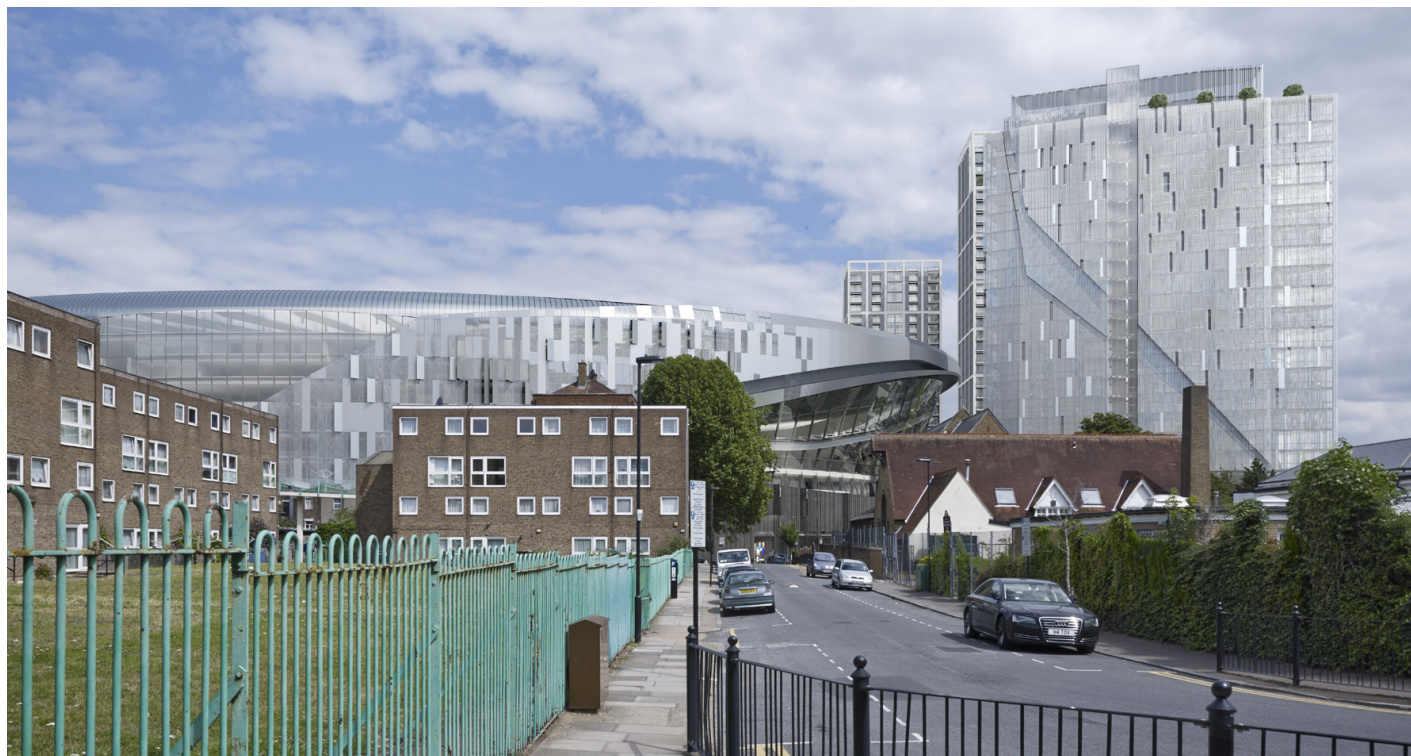
FIGURE 29. Brereton Road Looking East
